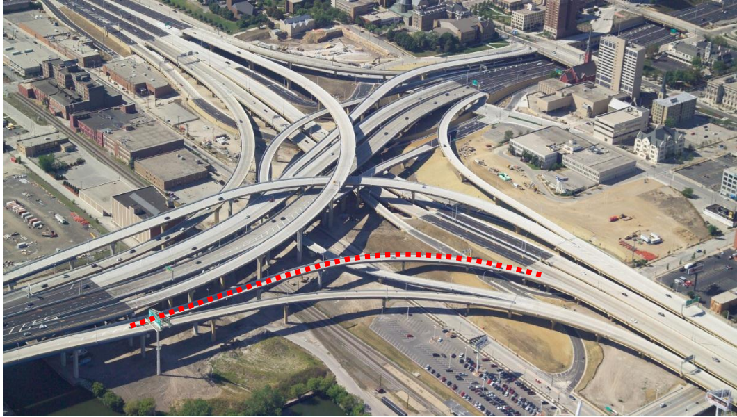
Figure 4.11. ETTTCR 15, Unit B-40-1122 of the Marquette Interchange, Milwaukee, WI. (Courtesy of T. Shkurti, HNTB).
