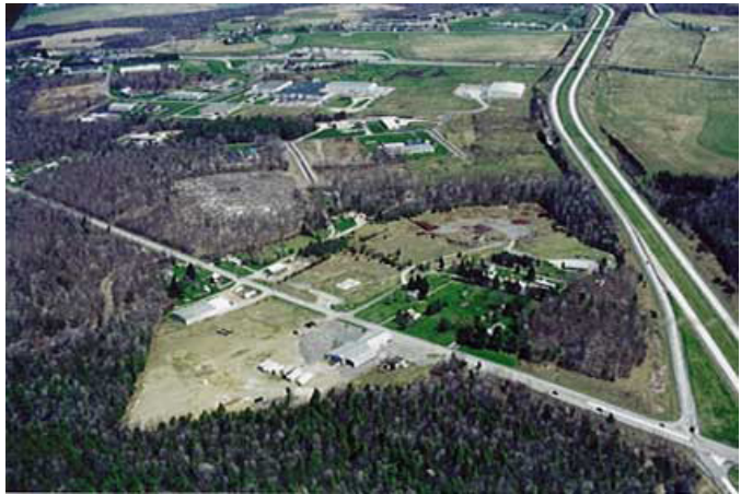
Figure 2.2.1 | View of Somerset Industrial Park Site
