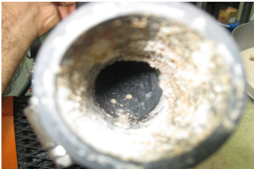
Figure 3.13: Material sticking to the walls of the feeder
