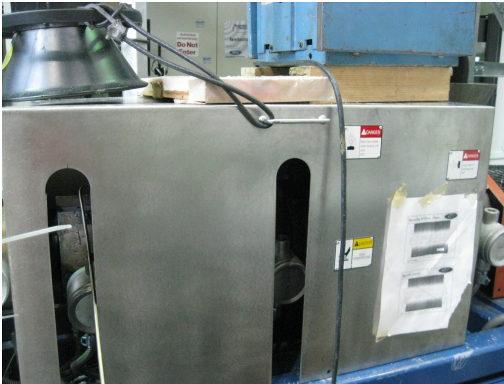
Figure 3.7: Stabilized cover to screw extruder
