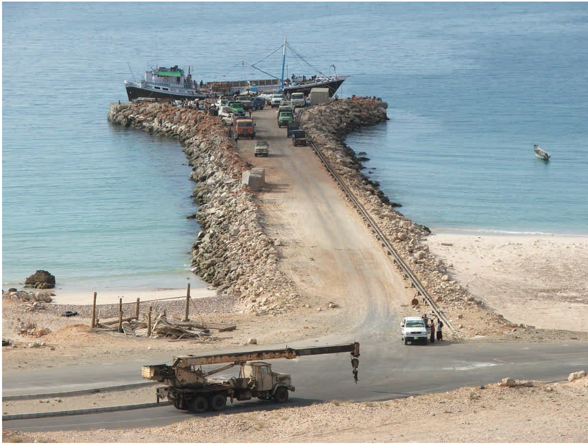
Figure 15 Jetty at Hawlaf with 4 lane highway access from Hadiboh, a typical wooden cargo vessel berthed alongside at the landing stage and a rusty crane as alternative to manual unloading – note the narrow beach to the west of the jetty and the wide beach to the east.
