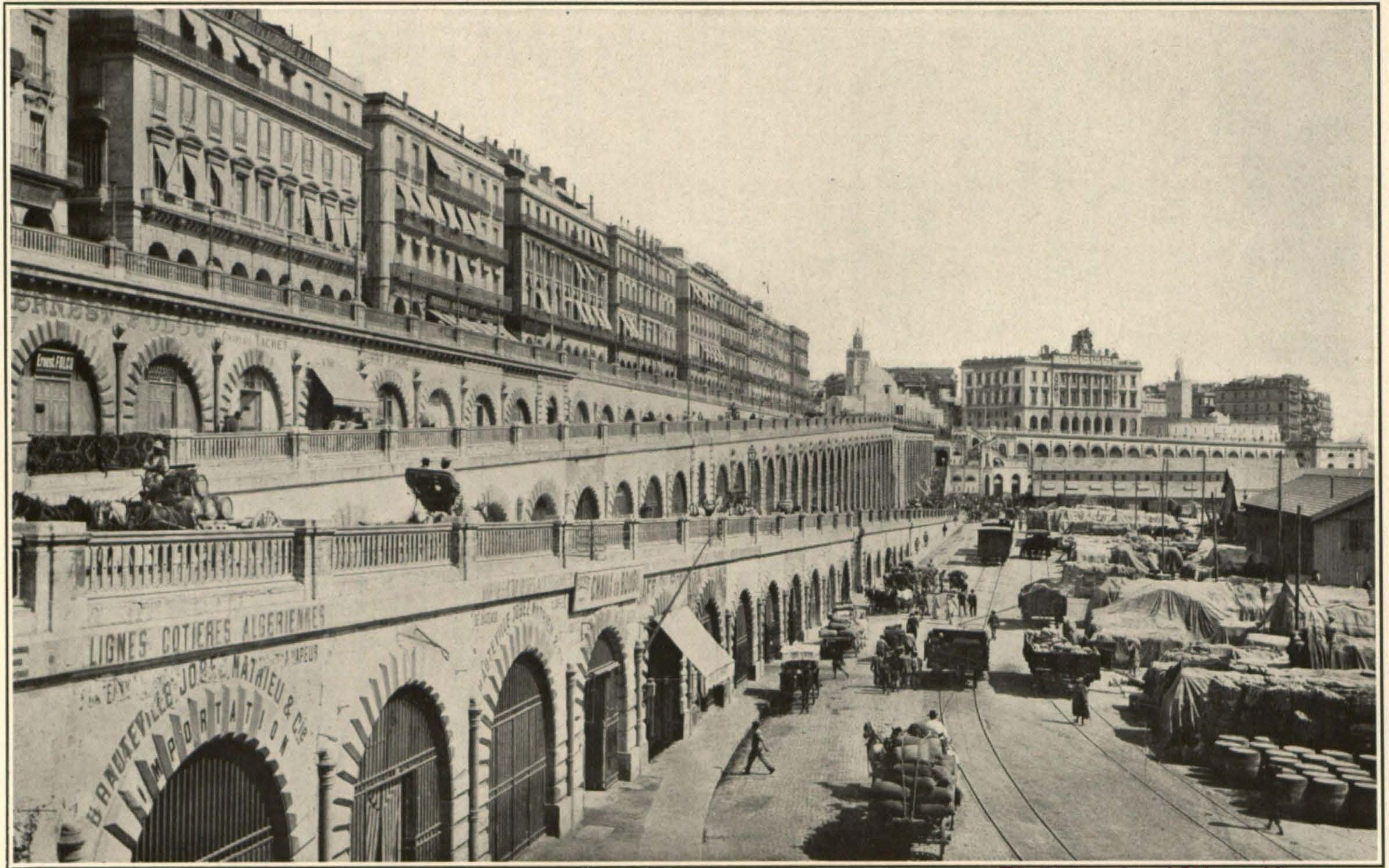
A CLOSER VIEW OF THE ALGIERS WATER FRONT. Showing the Storage Spaces Below the Esplanade and the Inclined Roadways.
