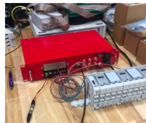
Figure 8: SAT-1 LS240 PSU (red box) undergoing testing. The LS240 PSU can be seen here connected to 1 LS240-2p and 3 LS240-8ps, replicating the experimental conditions for the SAT-1.
