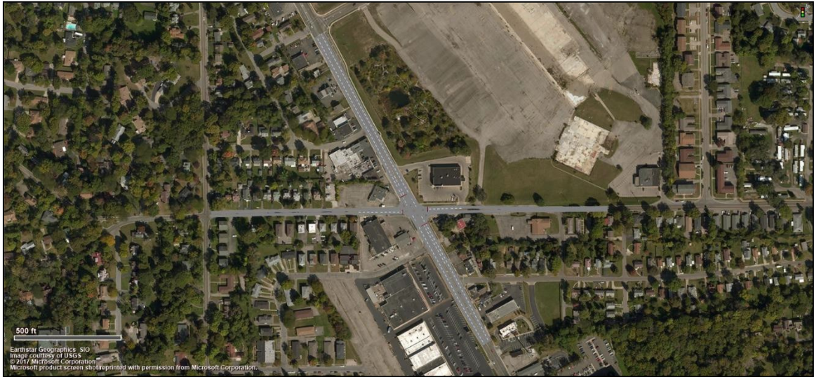
Figure C-1 N Main Street and Nottingham Road Intersection Layout and the Background Image in PTV Vissim
