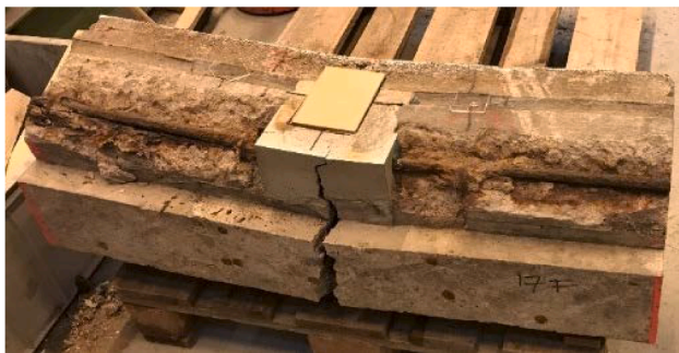
(c) Experimental crack pattern on the inner side, as measured.
