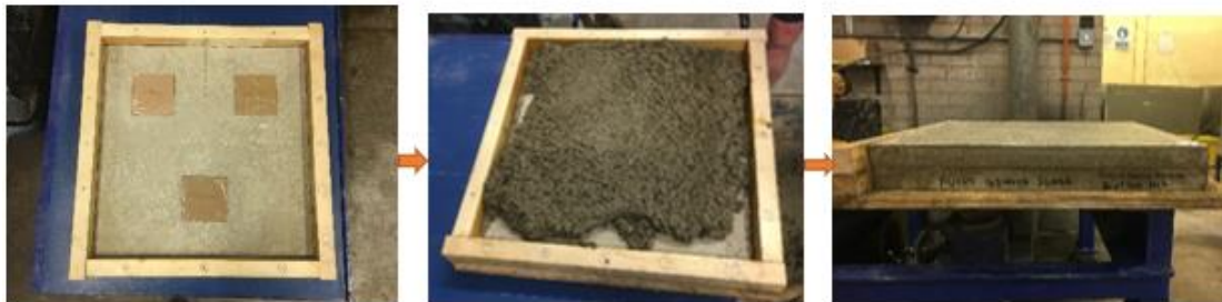
Figure 4-30: Casting of Two-slabs stacked system with three delaminations at the interface.
