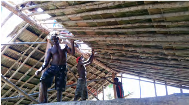
Figure 4: Villagers standing on the roof beams of a feast house installing palm leaf roofing panels over their respective clan hearths, in the village of Er, 2017. Image courtesy of the author. [Color figure can be viewed at wileyonlinelibrary.com ]
