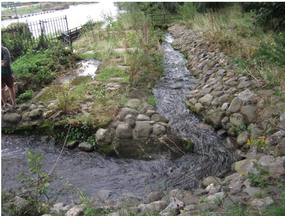
Figure 2.4: The semi-formalised nature-like bypass present at Naburn looking towards the downstream entrance for fish. The sluice is positioned immediately to the left of the image, out of shot.
