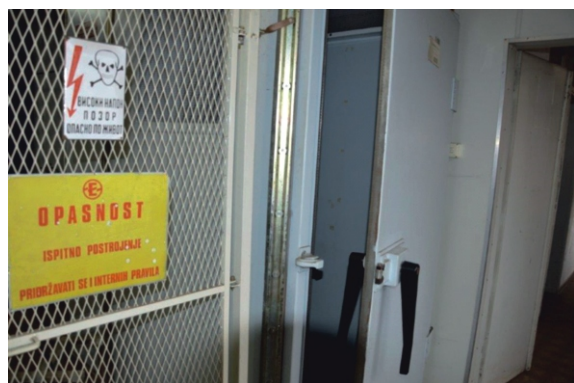
Figure 4. Commercial Faraday cage
