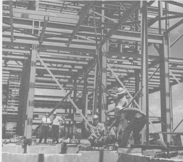
Construction in progress, Power and Recovery Boiler Building.
