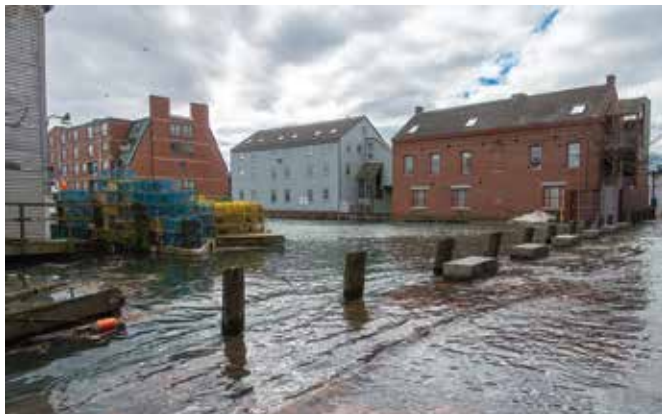
During the January 4, 2018 Nor'easter, powerful storm waves occurred at the same time as high tide. Water levels in Portland reached 13.8 feet, one of the three highest tides ever recorded. The tide remained above flood stage for nearly three hours, causing millions of dollars in damage statewide (Schmitt and Uteuova 2018).
