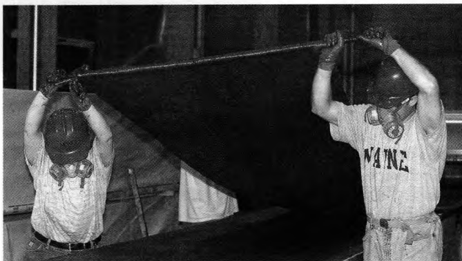
AEWC's Milbridge pier project
