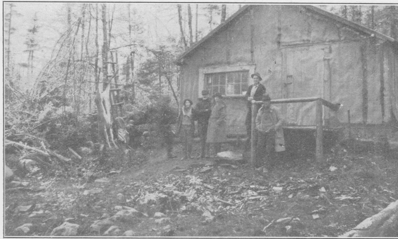
Construction Camp "Somewhere in Maine," where we spent the second night.
