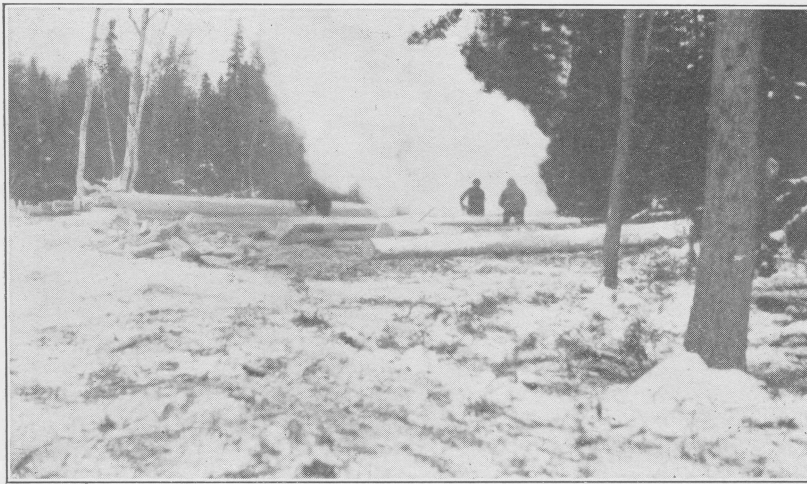
Hewing Timber for the Dam at McNally Pond, Machias Operation.
