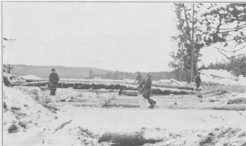
Putting in the Foundation of McNally Pond Dam, Machias Operation.
