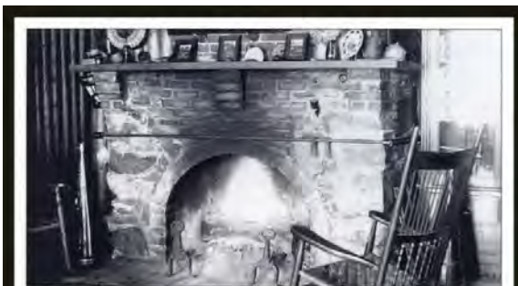
The Lakeside Camps, operated by N. W. McNaughton, were located on Schoodic Lake, famous for its large lake trout. This photograph shows one of the large fireplaces found here.
