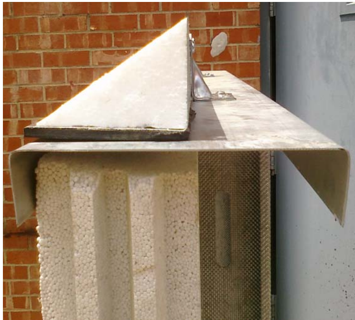
Figure 19: L-Joint fastened to ABT Panel During Fit Test
