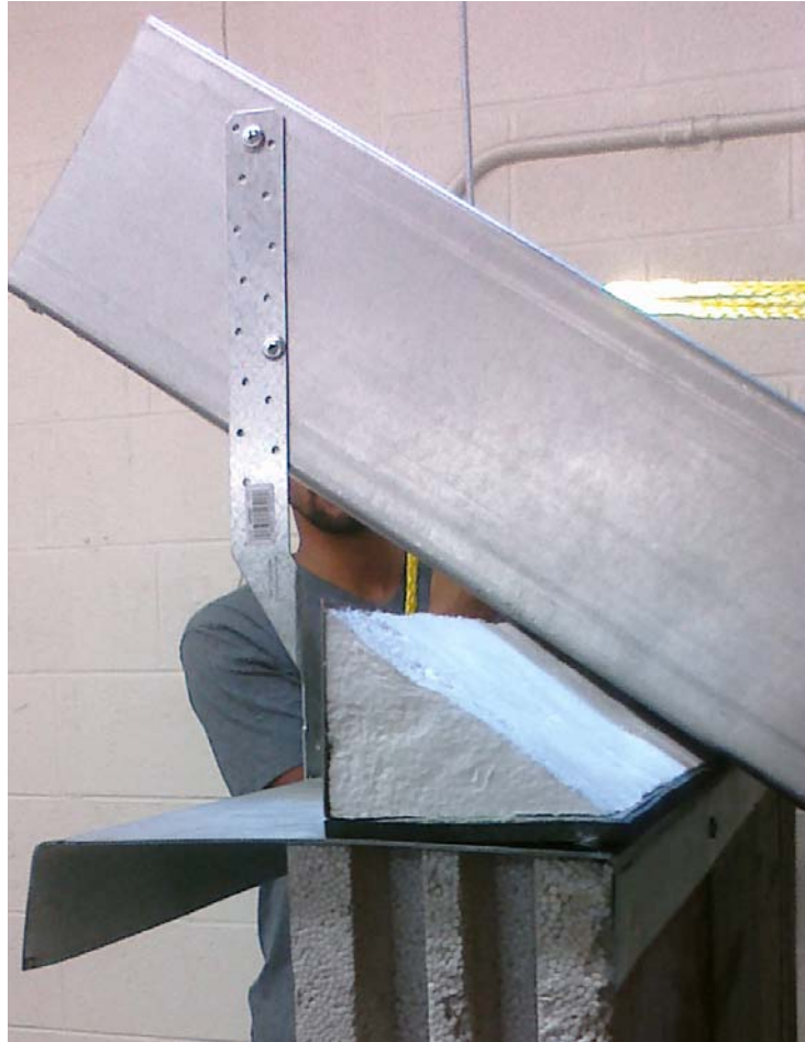
Figure 20: Assembly of L-Joint with Transcon Roof and ABT Wall Panel During Fit Test
