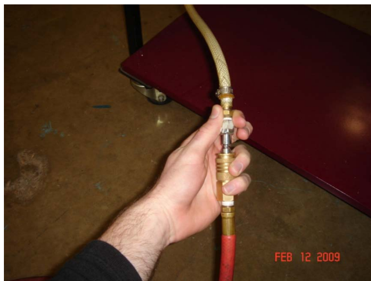
Figure 7. Connecting compressed air to system
