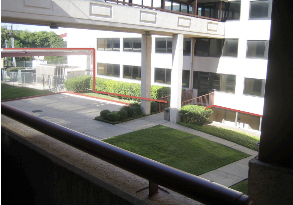
Figure F-2: Pipe Carrying Condensate Water to Cooling Tower
