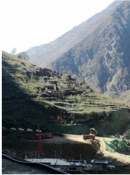
Figure 25: Ruins of the destroyed village above Baijiaduo
