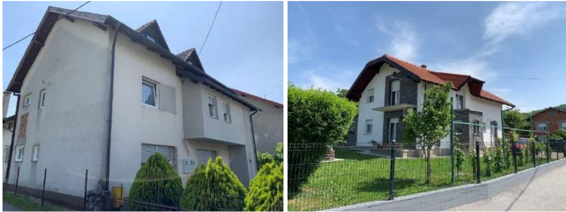
Figure 5-42: RC buildings mistakenly reported as masonry
