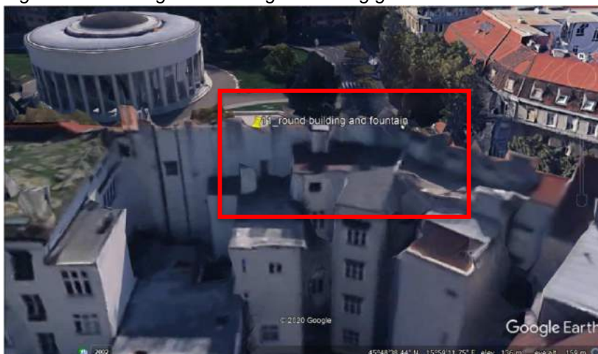
Figure 5-12 – Google Earth image indicating gable failure
