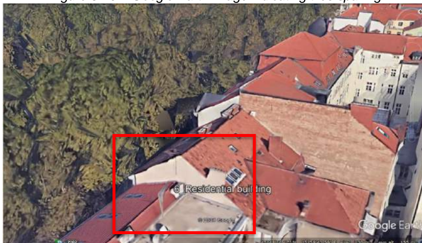
Figure 5-11 – Google Earth image indicating gable failure
