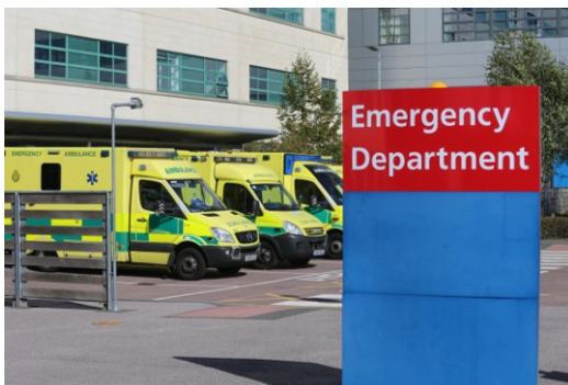
Figure 2.3.2: Hospital emergency department (©Stuart Harrison).
