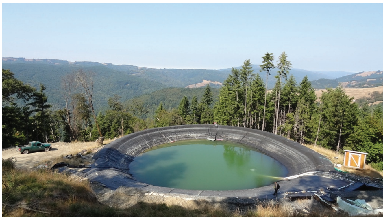
Figure 3. An illegally constructed pond and water diversion associated with a marijuana cultivation site in northern California. Photograph: Scott Bauer.
