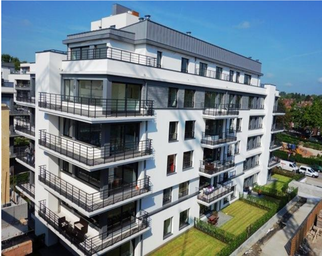
Picture 3.7.4-1: Block 1 building completed
