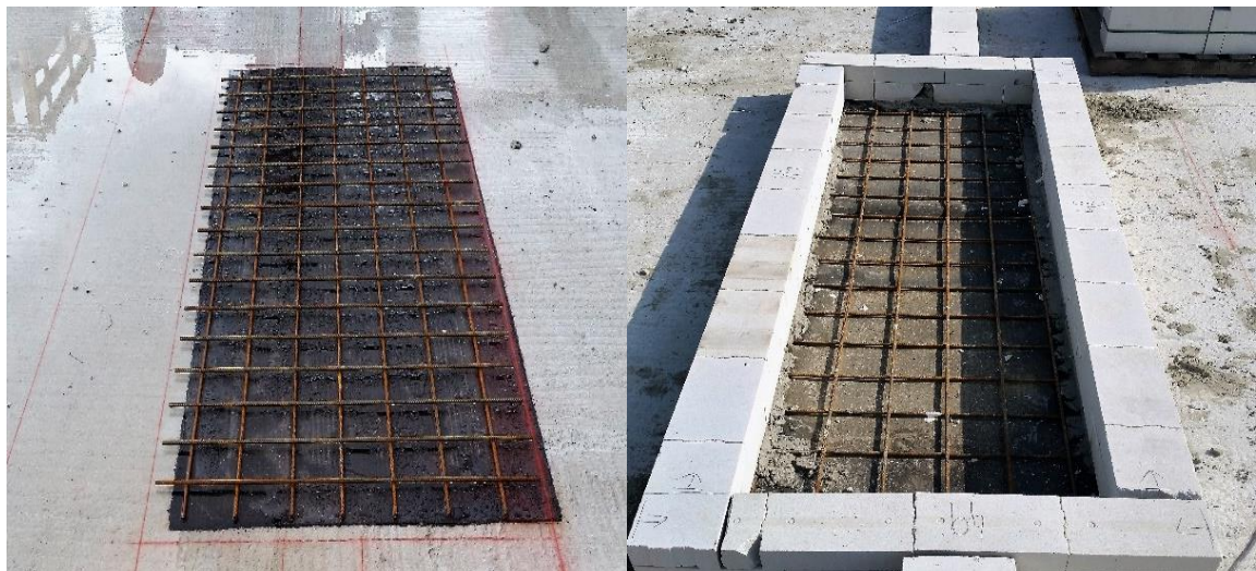
Figure 6.5.6-1 Steps 1 to secure the works in the raisers of block 2
