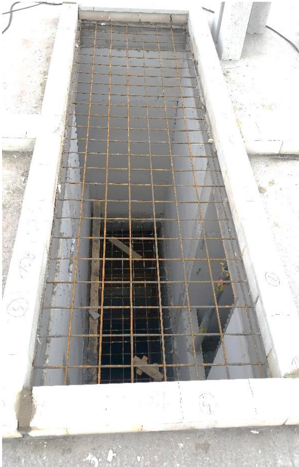
Figure 6.5.6-3 Step 3 to secure the works in the raisers of block 2
