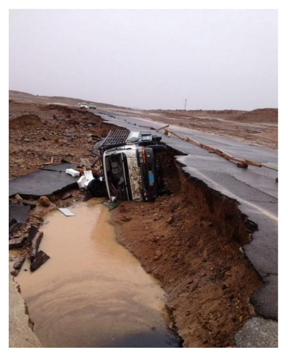
Figure 4.15 Road collapse and one vehicle was sent off the road after intense rainstorm (01/18/2010).
