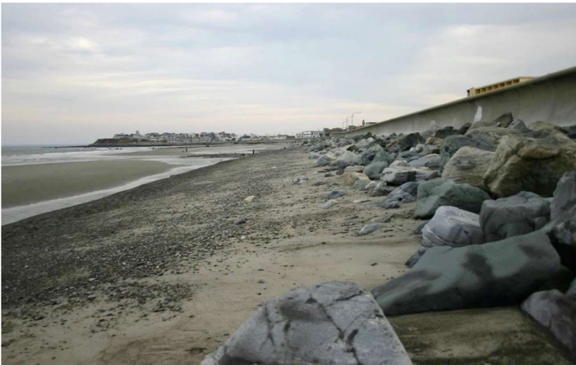
Figure NB-10. North Beach looking south from station NB03 on April 11 (left photograph) and on a foggy day in September 19, 2017 (right photograph). In April the beach was highly eroded and the low tide terrace (lower beach) elevation was much lower than September. A sand ramp is also visible in April adjacent to the seawall, which can form during storms by scouring the lower beach and transporting the sand landward. In September the beach had regained elevation through deposition of a sand wedge that buried the pebble lag seen in April.
