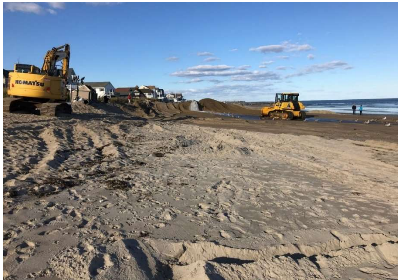
Figure SB-7. Beach nourishment on Seabrook Beach on October 26, 2019. The sand was pumped onto the beach and then distributed by a power shovel, bulldozer, and ultimately natural processes.
