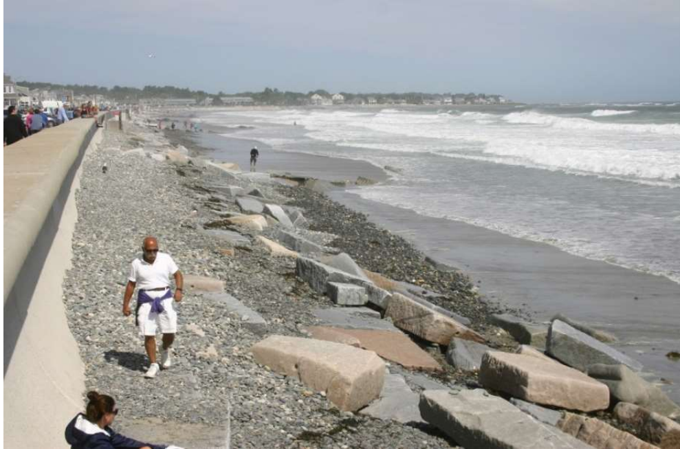
Figure NB-5. During storm conditions waves push gravel up the beach and often form gravel ramps as shown in this photograph taken on September 5, 2016.
