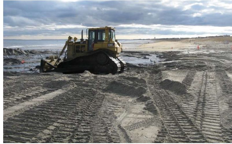
Figure 4-2. Beach nourishment at Seabrook Beach using dredged material from Hampton-Seabrook Harbor (December 11, 2012). The sand was pumped onto the beach via a pipeline (left photograph) and then graded with a bulldozer (right photograph).
