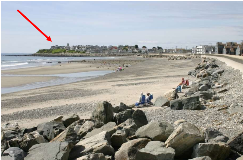
Figure NB-3. North Beach looking south on June 6, 2019. Great Boars Head (arrow) forms its southern boundary. A cement seawall extends the entire length of the beach. Note the riprap at the base of the seawall placed to diminish wave impact and the megaclast platform.
