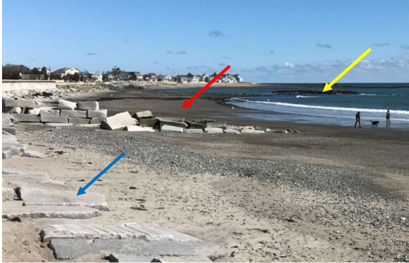
Figure NB-2. Photograph of the northern headland at North Beach taken on March 18, 2017 from station NB01. Note the stone groin in the foreground (red arrow), stone blocks at the base of the seawall (blue arrow), and a megaclast platform at the northern end of the beach (yellow arrow).
