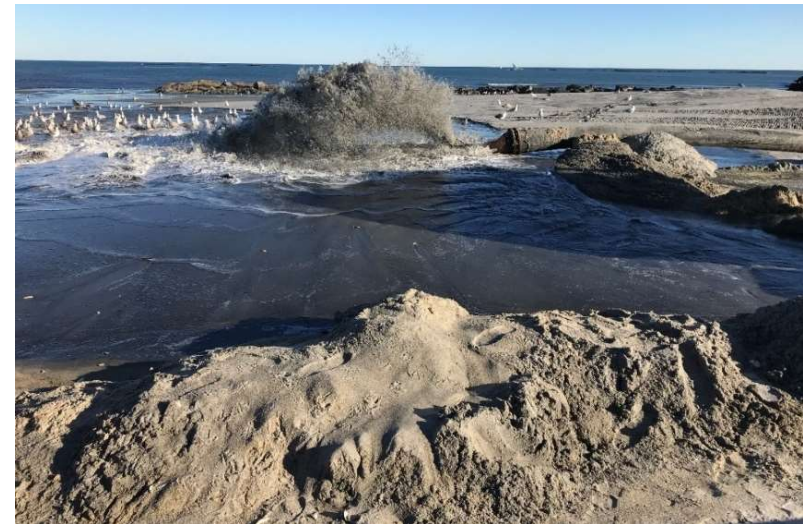
Figure 4-3. Beach nourishment at Hampton Beach State Park using dredged material from Hampton-Seabrook Harbor (November 23, 2019). The sand was pumped onto the beach via a pipeline (left photograph). Photograph on the right is a close-up of sand discharged from the pipe.
