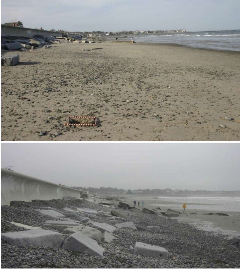
Figure NB-11. North Beach looking north from station NB02 on April 11 (upper photograph) and September 19, 2017 (lower photograph). The gravel ramp seen in September is covered with sand in April which is atypical for NH beaches. Normally, the gravel ramps are more exposed in winter. However, this does not represent accretion of the beach. Rather the lower beach was scoured by winter storms in April and the sand pushed up to the seawall (see Figure NB-8a).
