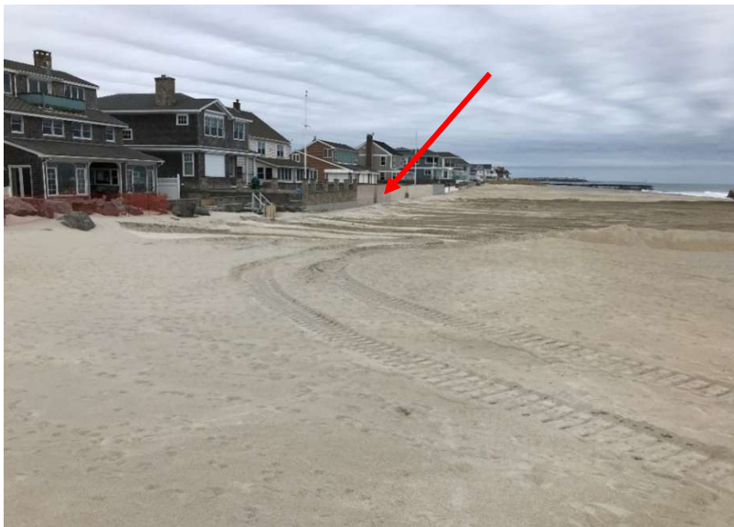
Figure SB-3. Homes north of the major dunes on Seabrook Beach are typically protected by a seawall (arrow) as shown in this photograph from February 4, 2020. Sand dredged from Hampton and Seabrook Harbor was placed on the beach in late fall 2019.
