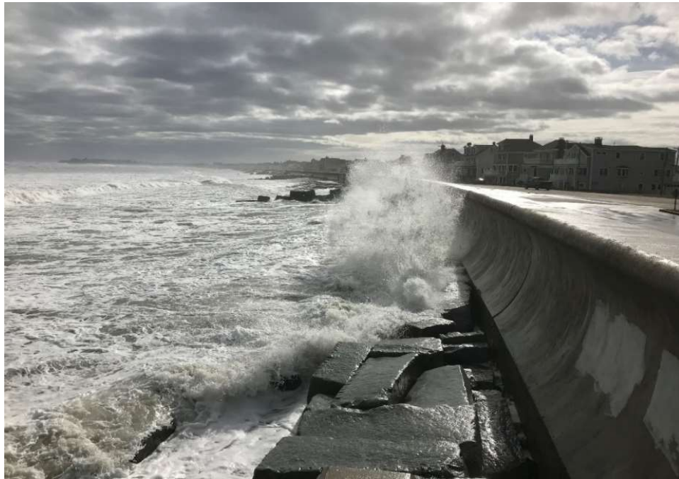
Figure NB-7. Storm waves following the nor'easter Riley at North Beach. The low elevation of the beach along with the storm conditions resulted in the seawall being impacted by waves. The photograph was taken on March 3, 2018 after the peak of the storm and the largest waves.
