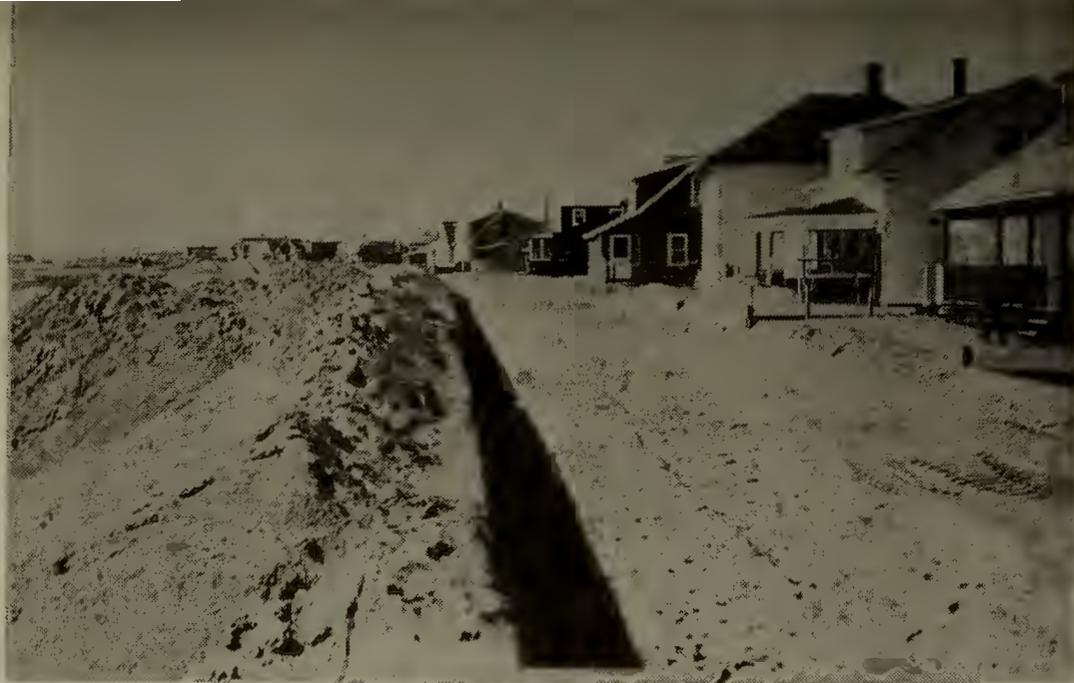
Figure 17. February Blizzard of 1978 caused 25000m<sup>3</sup> of sand to be transported over the seawall along Yirrell Beach.
