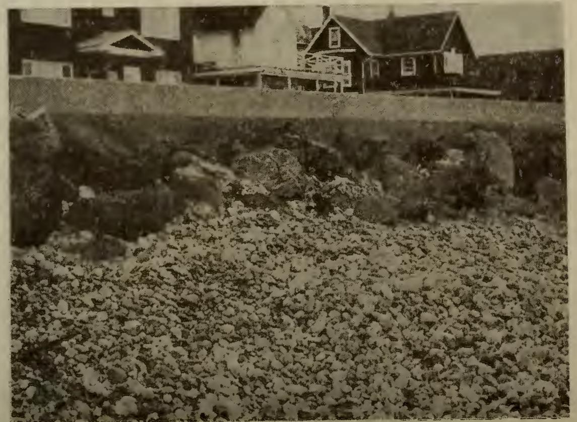
Figure 35. Gravel that had accumulated around riprap.
