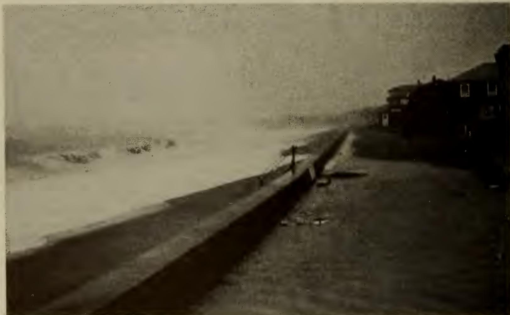
Figure 16. Ground photograph taken during the 25 January 1979 northeast storm. Waves are eroding the beach face and depositing some of the sediment next to the seawall.
