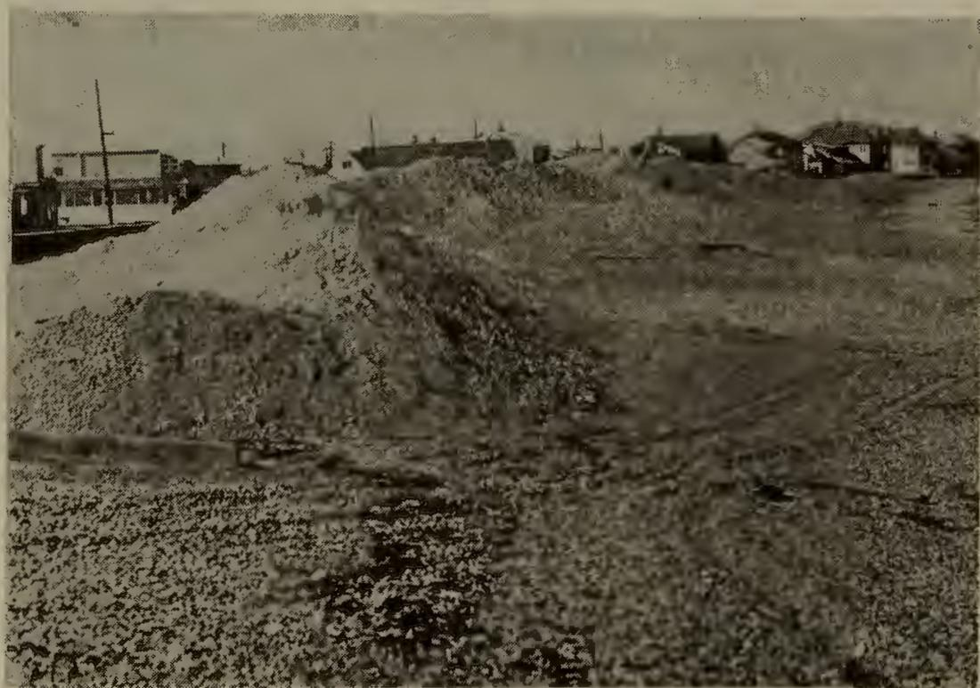
Figure 18. An artificial dune ridge was constructed from the sand removed from behind the seawall along Yirrell Beach after the February Blizzard.
