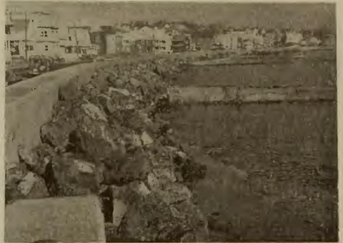
Figure 34. Riprap along northern Winthrop Beach. Photograph taken right after completion of project.
