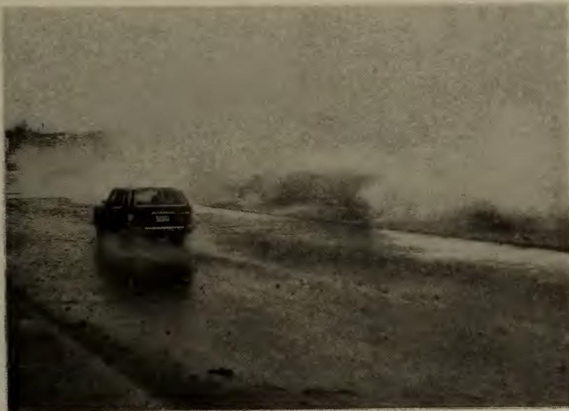
Figure 36. Photograph of water and gravel being transported over the seawall after the seawall had been riprapped.
