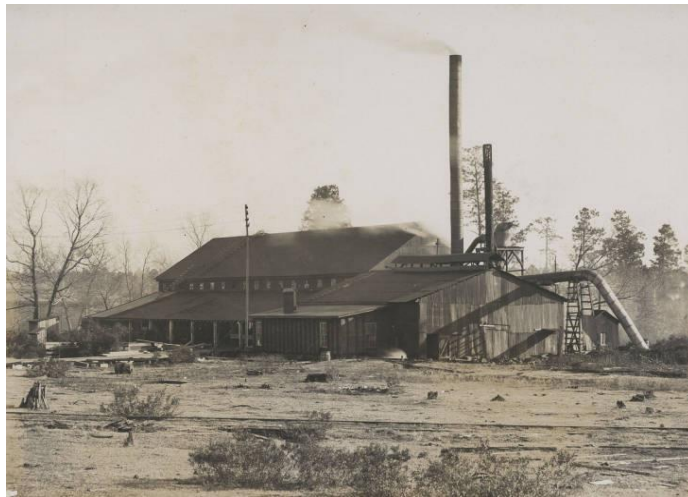
Exhibition Text: Thompson and Tucker Lumber Company Mill, Willard, TX, 1890s. Lumber mills and the lumber industry are still, and always have been vital to the economy of East Texas.
