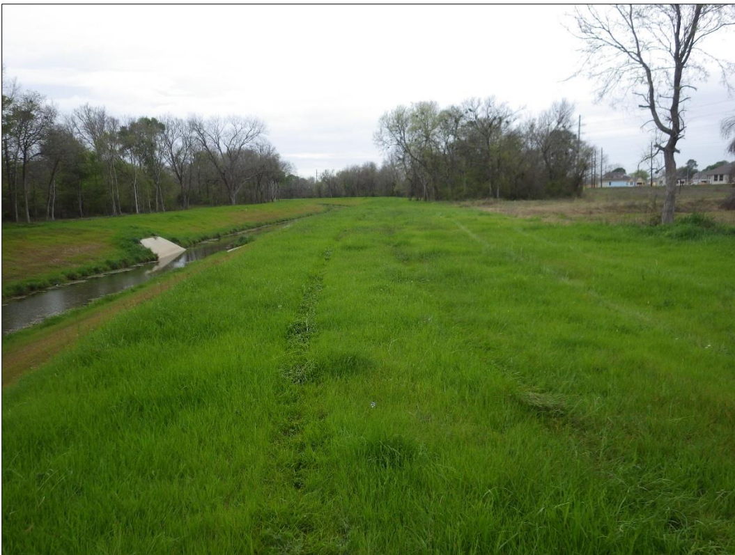
Figure 7. Channelized Seabourne Creek showing maintained creek bank.
