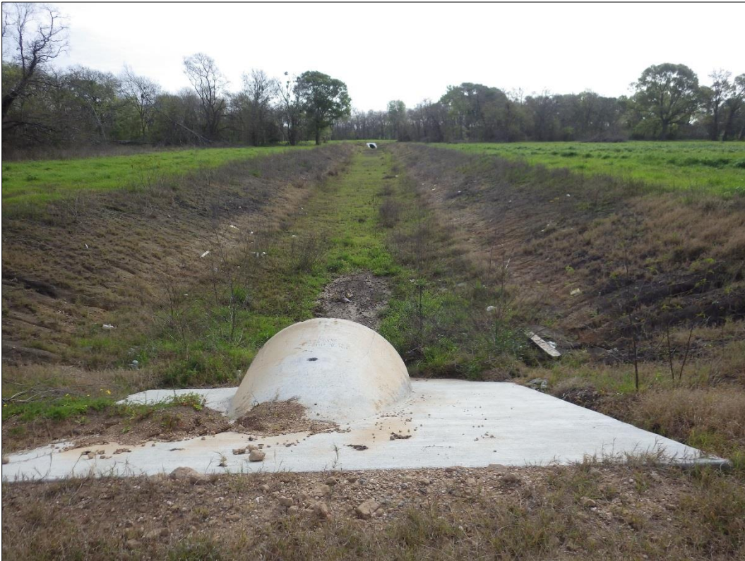
Figure 6. Excavated drainage ditch through Parcel 1.
