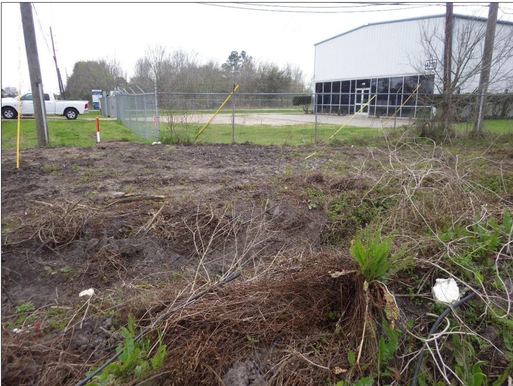
Figure 9. Cleared area for utilities at the eastern end of Parcel 2.
