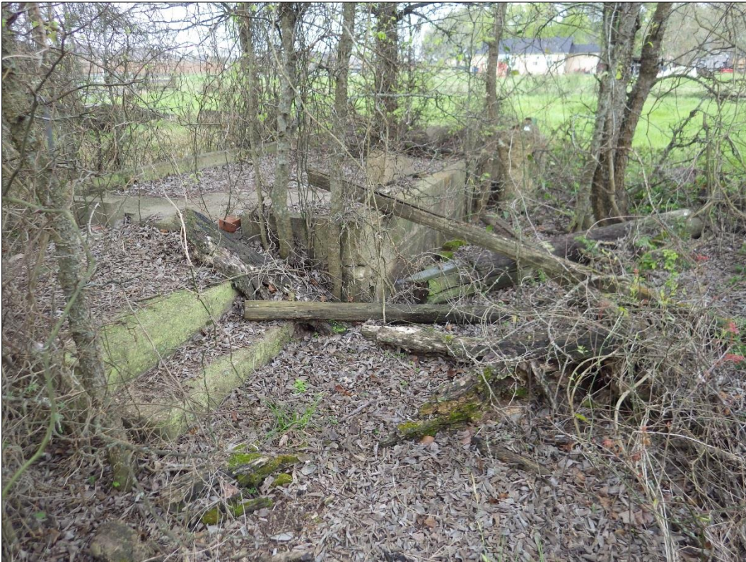
Figure 18. Foundation remains of house in site 41FM363.
