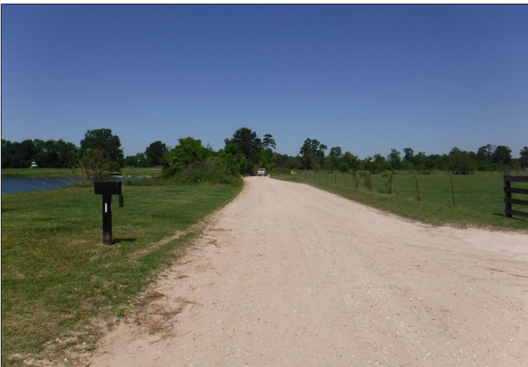
Figure 7. Existing Old Spanish Trail Right-of-Way (Facing Northwest)
