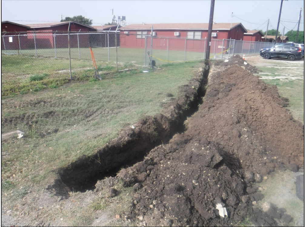
Figure 5-8. Overview of the western APE excavations, facing southwest.
