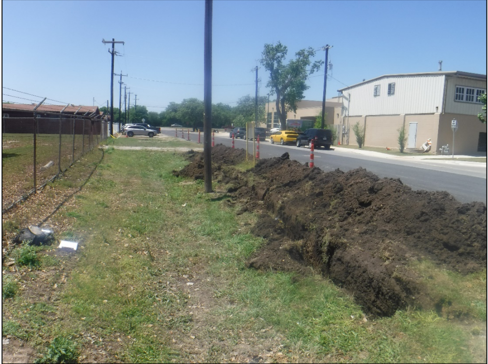
Figure 5-4. Overview of central APE trench, facing west.
