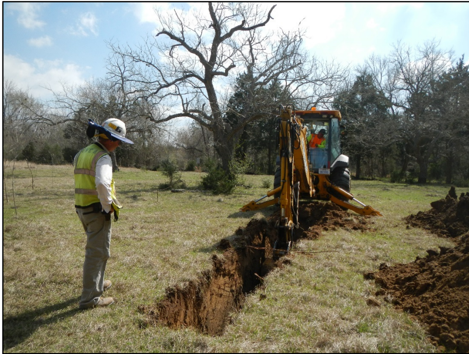
Figure 4. Backhoe trench BHT01 overview, facing east.
