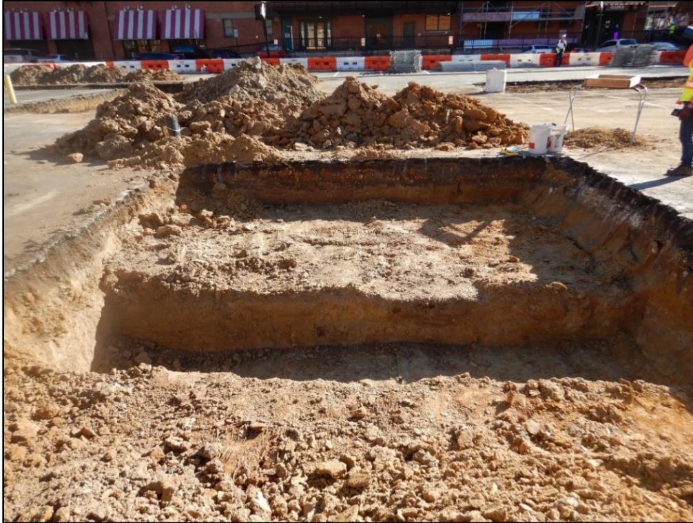
Figure 19. Block A, showing Trench 1; view facing south.
