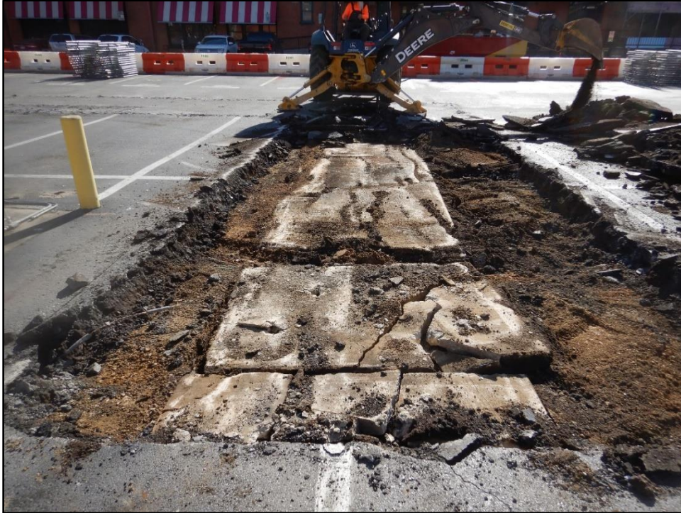
Figure 26. Concrete walkway (Feature 1) found in Block C. View facing south.
