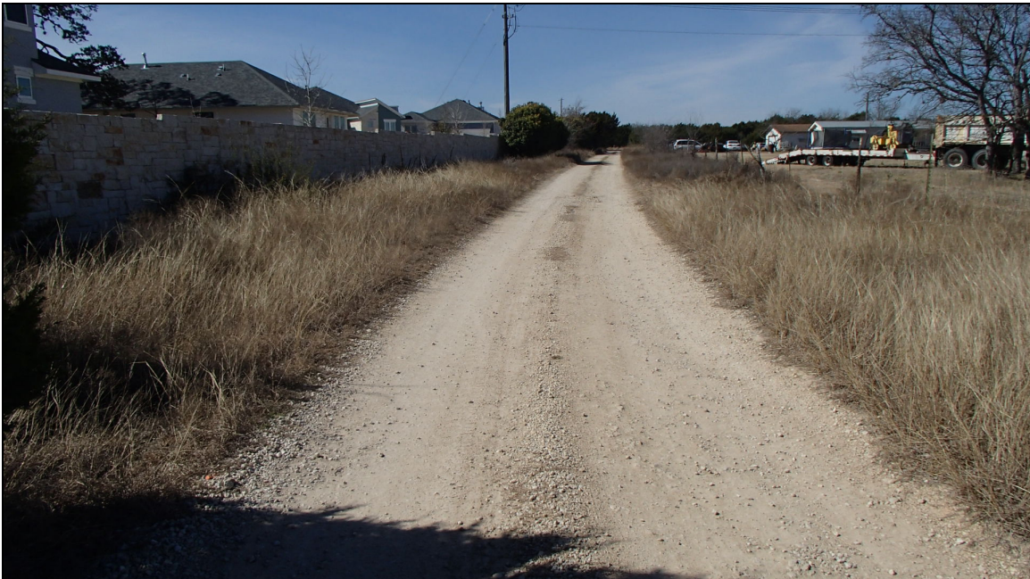
Figure 8. North end of alignment showing residential area, facing west
