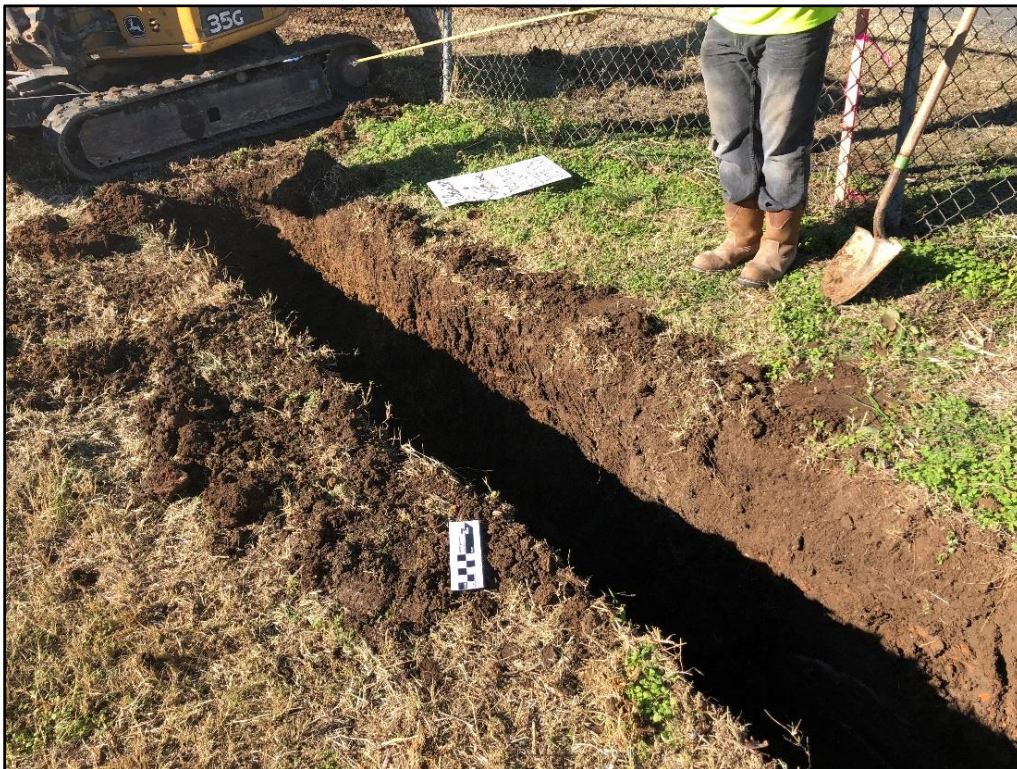
Figure 5-6. Overview of linear trenching excavations, facing north.
