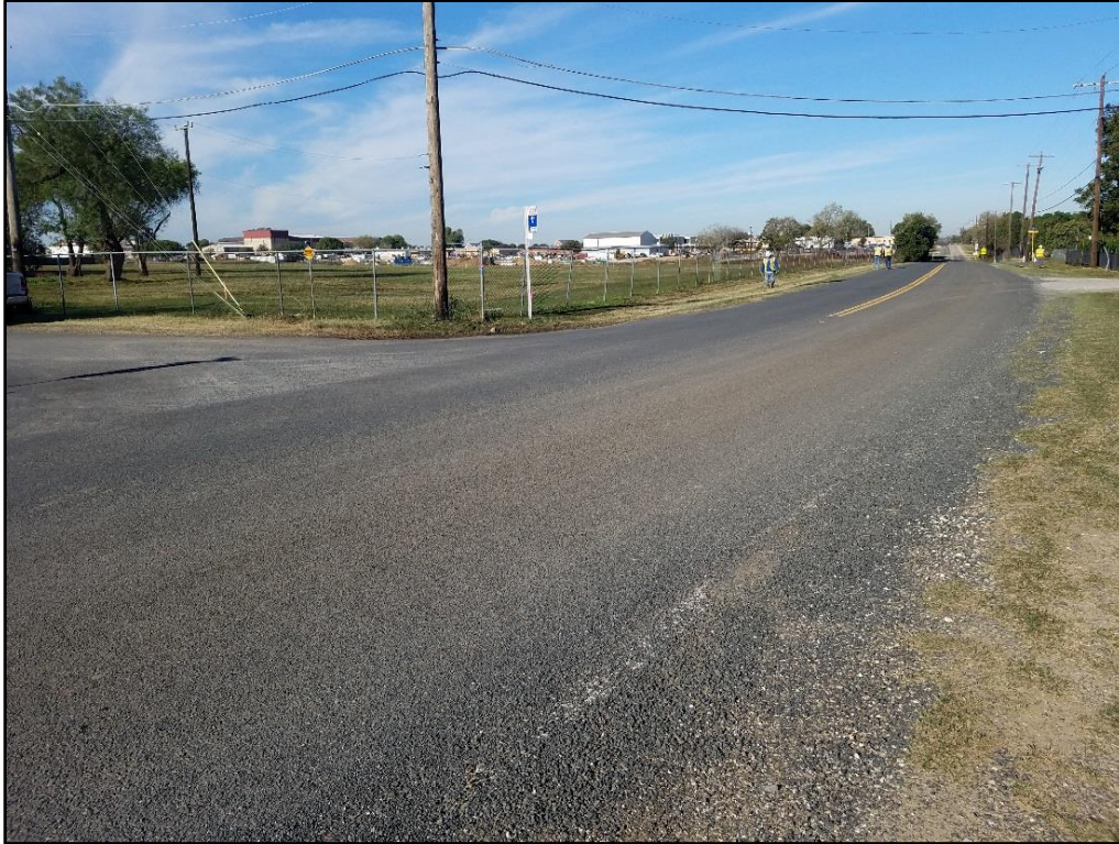
Figure 5-2. Overview of APE with Southside High School campus in background, facing west.
