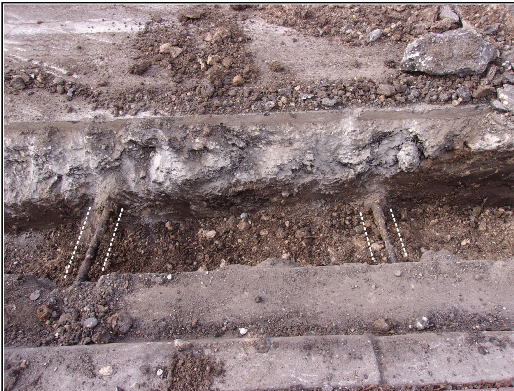
Figure 4-3. Utility pipes within monitored trench. Dotted white lines illustrate pipes.
