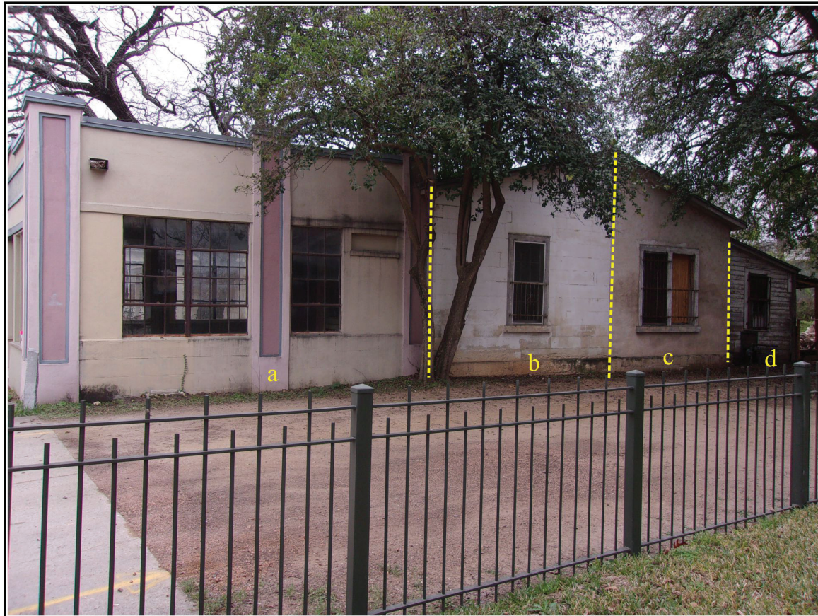
Figure 3-2. 1009 S. Alamo Street. Yellow delineates separate construction episodes. Section b appears to be original limestone construction; a , c , and d are likely later additions.
