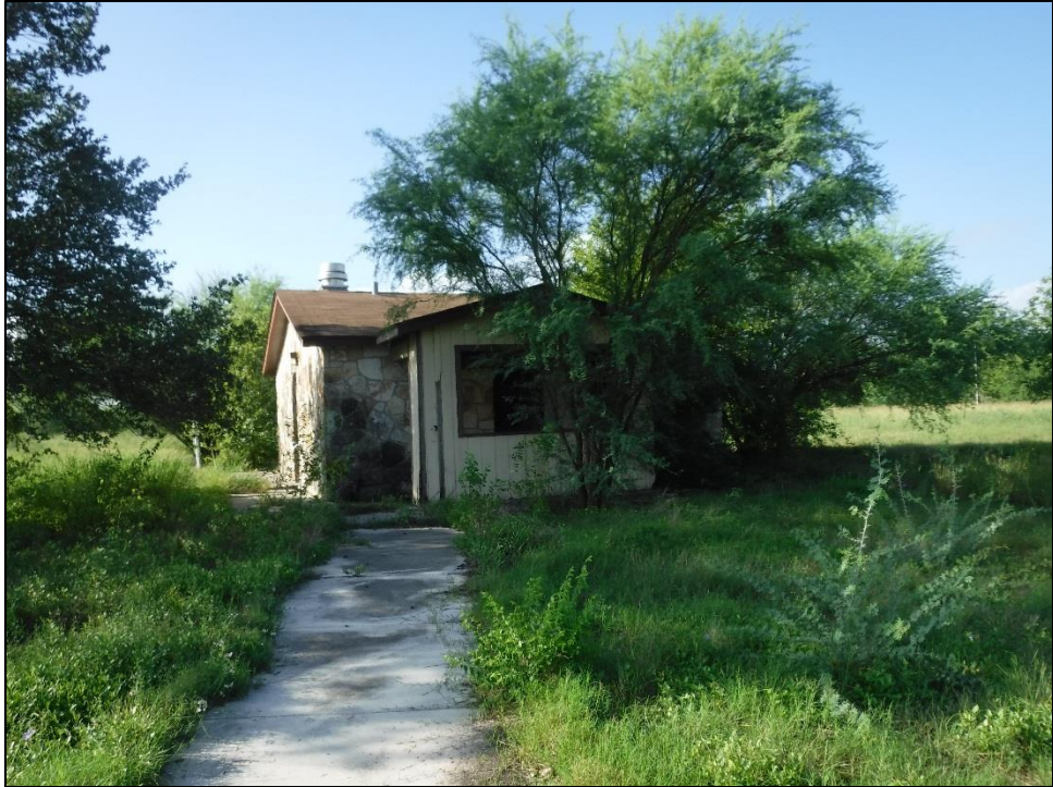
Figure 5-2. FamCamp Restroom and Showers, facing north.
