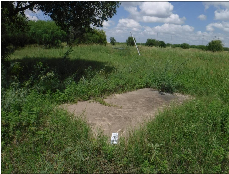
Figure 5-8. Cement Pad 2, facing north.
