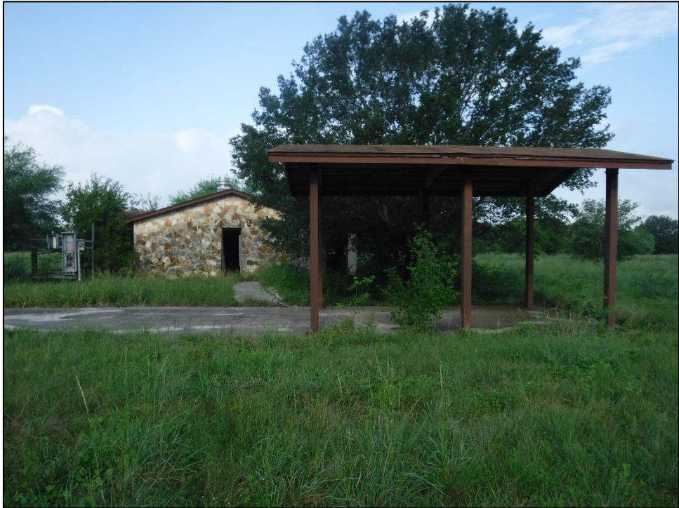
Figure 5-3. Covered concrete slab, facing west.
