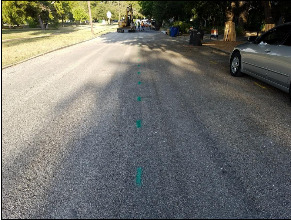
Figure 5-1. Overview of the APE with new sewer main marked in green, facing west.
