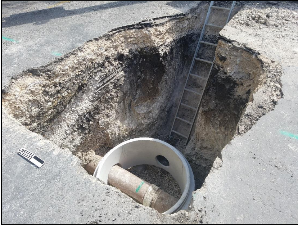
Figure 5-3. Installation of new sewer manhole at the junction of an existing SAWS sewer main, facing northeast.
