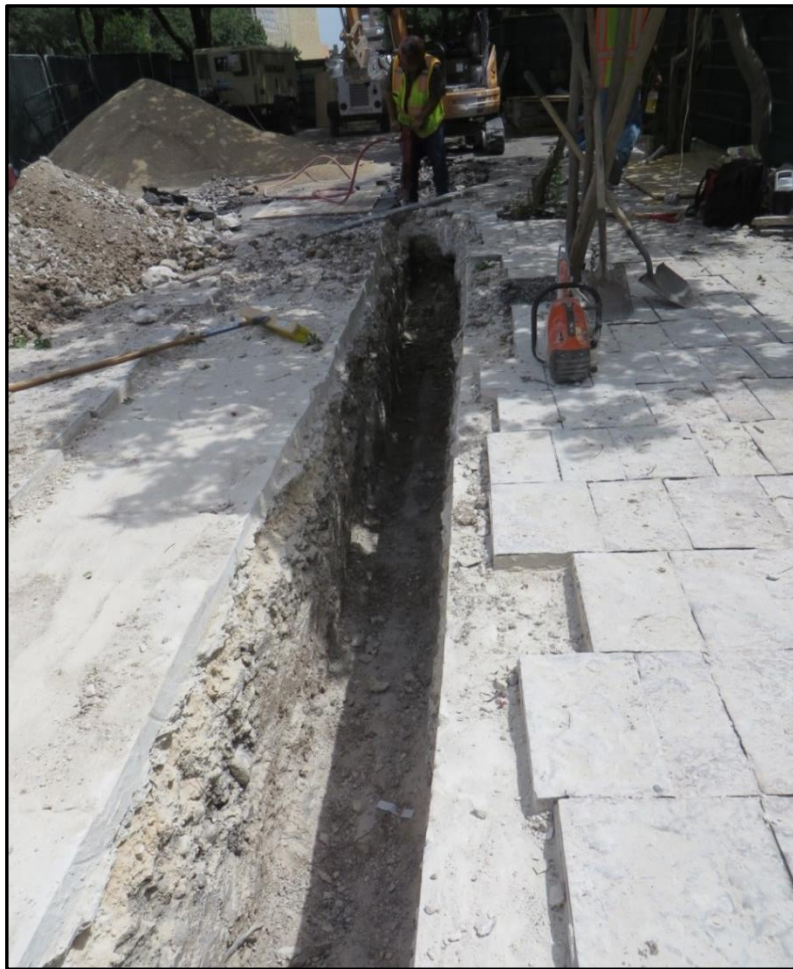
Figure 4-5. Use of the impact hammer. Portion of the Phase II trench, facing south.
