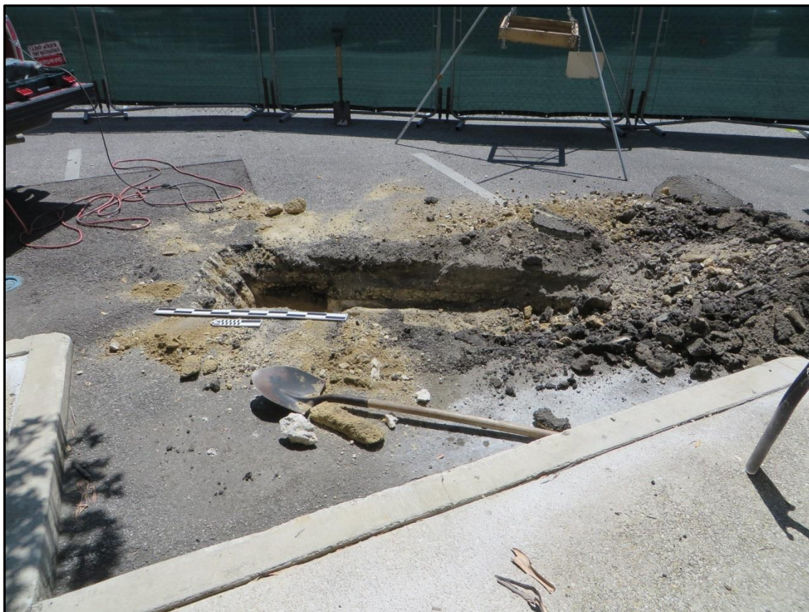
Figure 4-2. The RKEI exploratory trench in Phase I.
