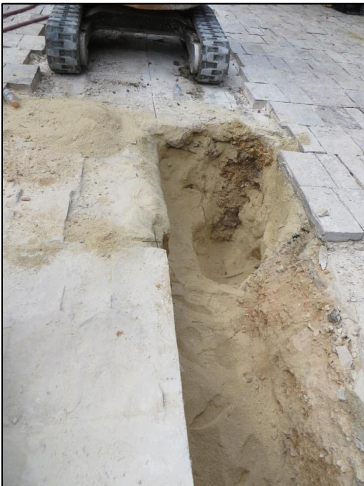
Figure 4-6. Phase II trench showing sand and water line servicing the Spanish Governor's Palace.
