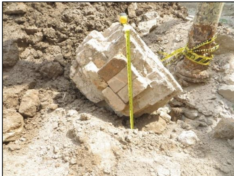
Figure 14. A portion of the removed brick and mortar, 75 cm in length.
