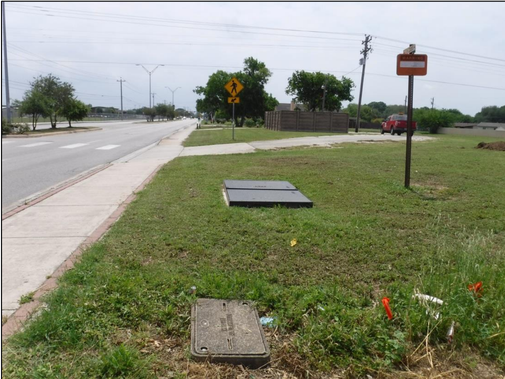
Figure 5-5. Utilities along Schertz Parkway, within the northeast corner of the Area of Potential Effects; facing southeast.
