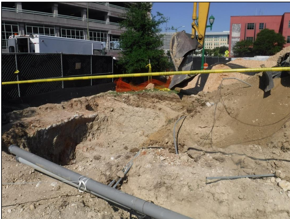
Figure 5-17. Showing orientation of T-5 with T-4, facing southwest.
