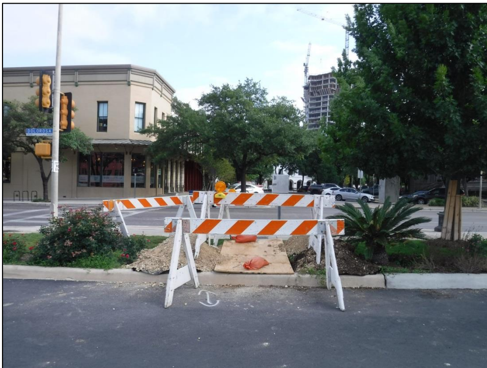
Figure 5-3. Overview of BP1, facing north.
