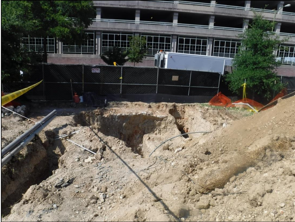
Figure 5-15. Overview of T-3 and T-4, facing south.
