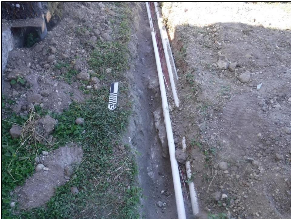
Figure 5-11. Limestone in the northern portion of T-2, facing south.
