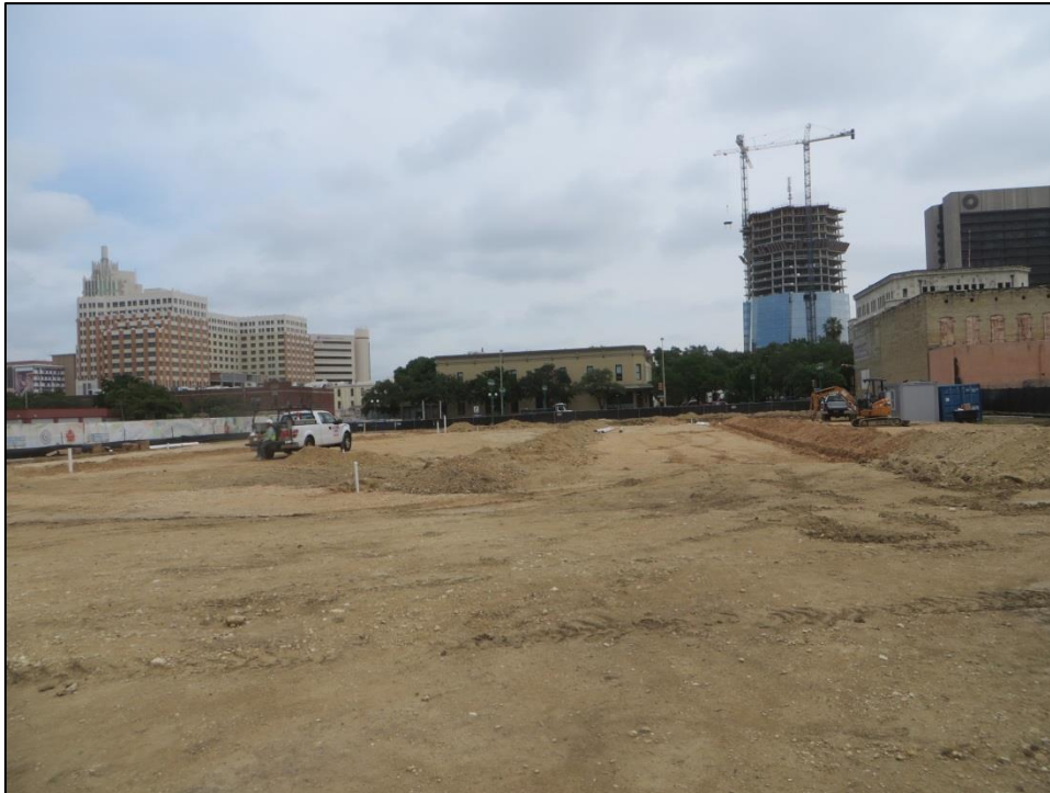
Figure 5-2. Overview of Project Area, facing north.
