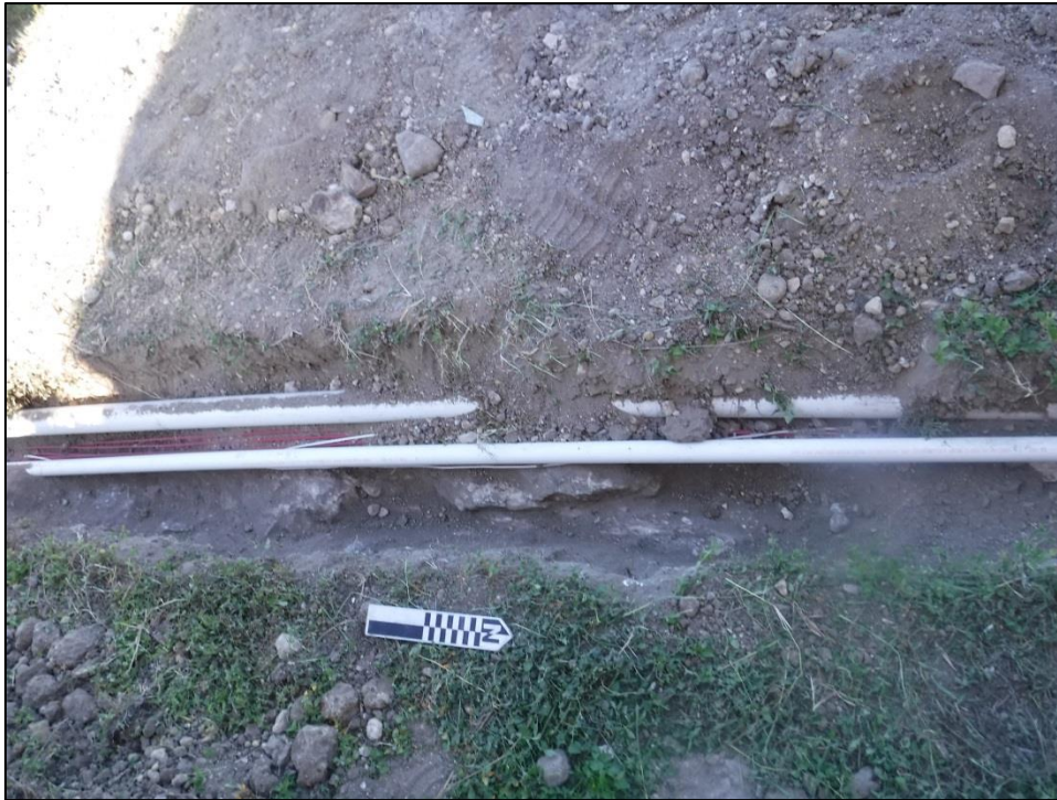
Figure 5-12. Limestone in the northern portion of T-2, facing west.
