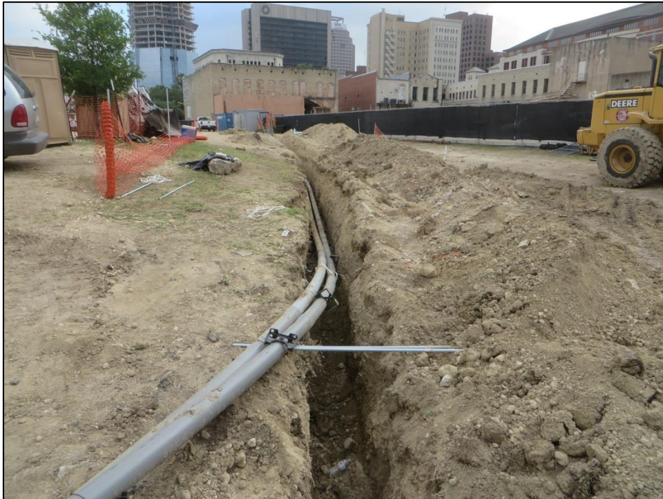
Figure 5-16. View of T-5 with pipes installed, facing north.
