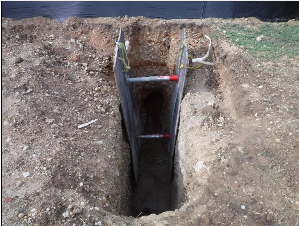
Figure 5-13. T-3 with shoring placed in trench, facing south.
