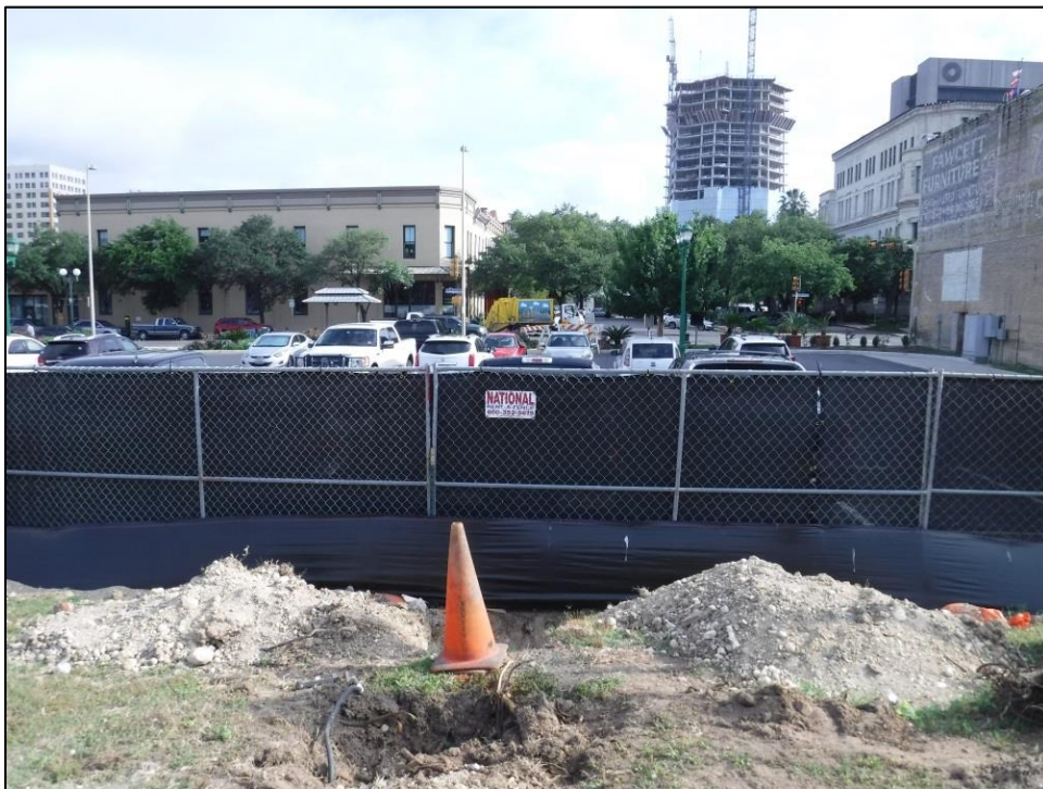
Figure 5-6. Overview of BP2, facing north.
