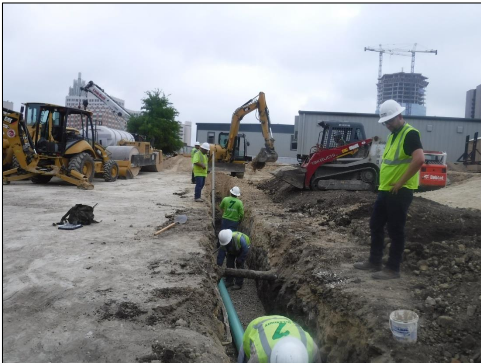
Figure 5-27. Crew excavating T-8, facing north.
