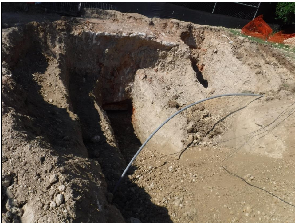
Figure 5-14. View of T-4, facing southwest.
