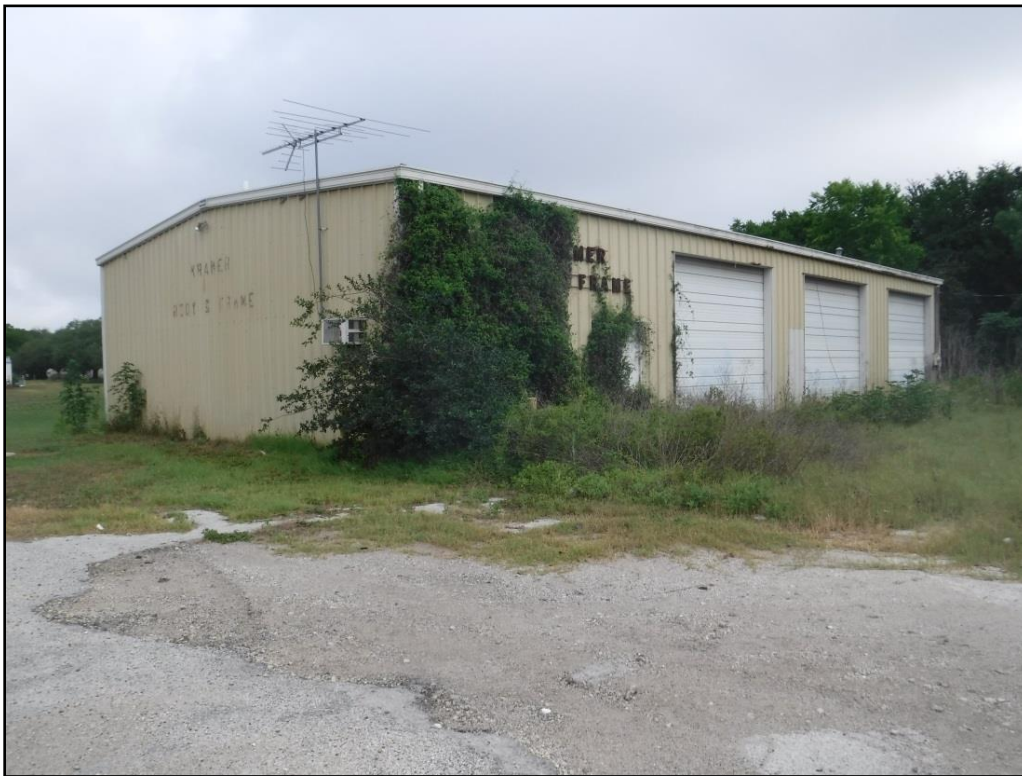
Figure 5-39. Southeastern and southwestern elevations of Historic Resource 1, facing north.
