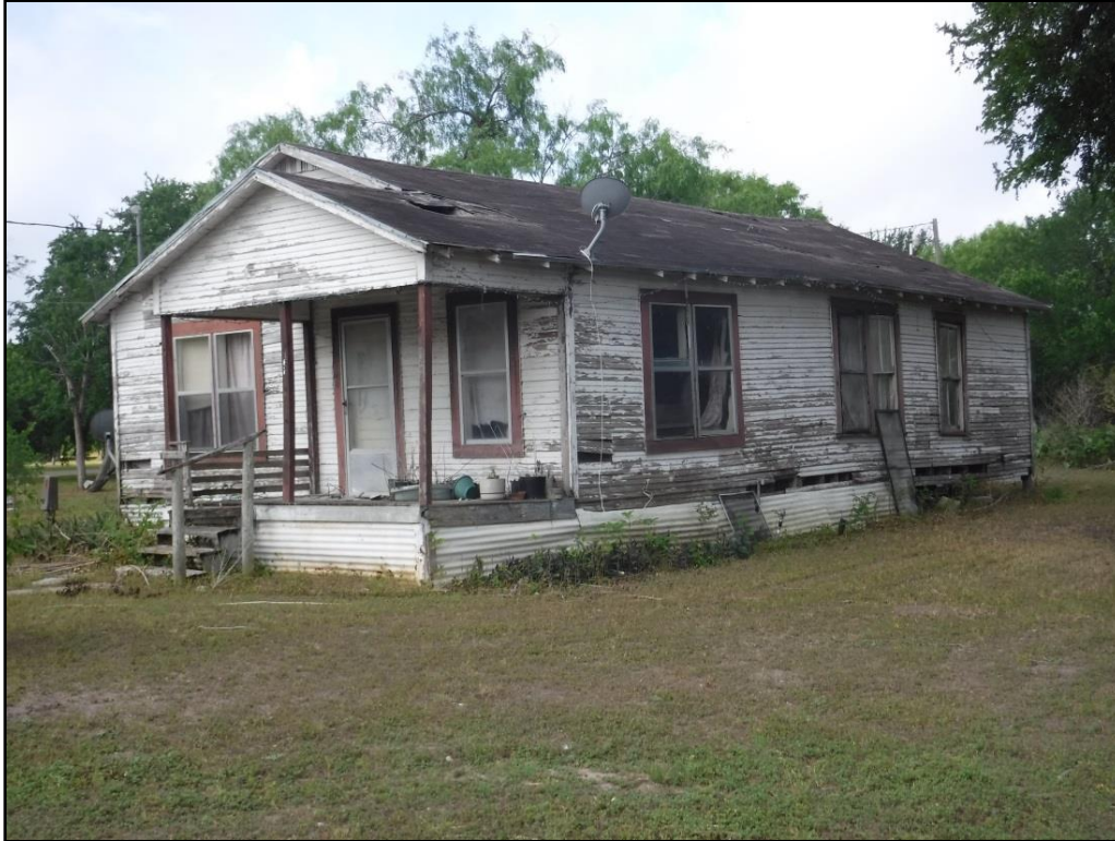
Figure 5-45. Northwestern and northeastern elevations of Historic Resource 4, facing south.
