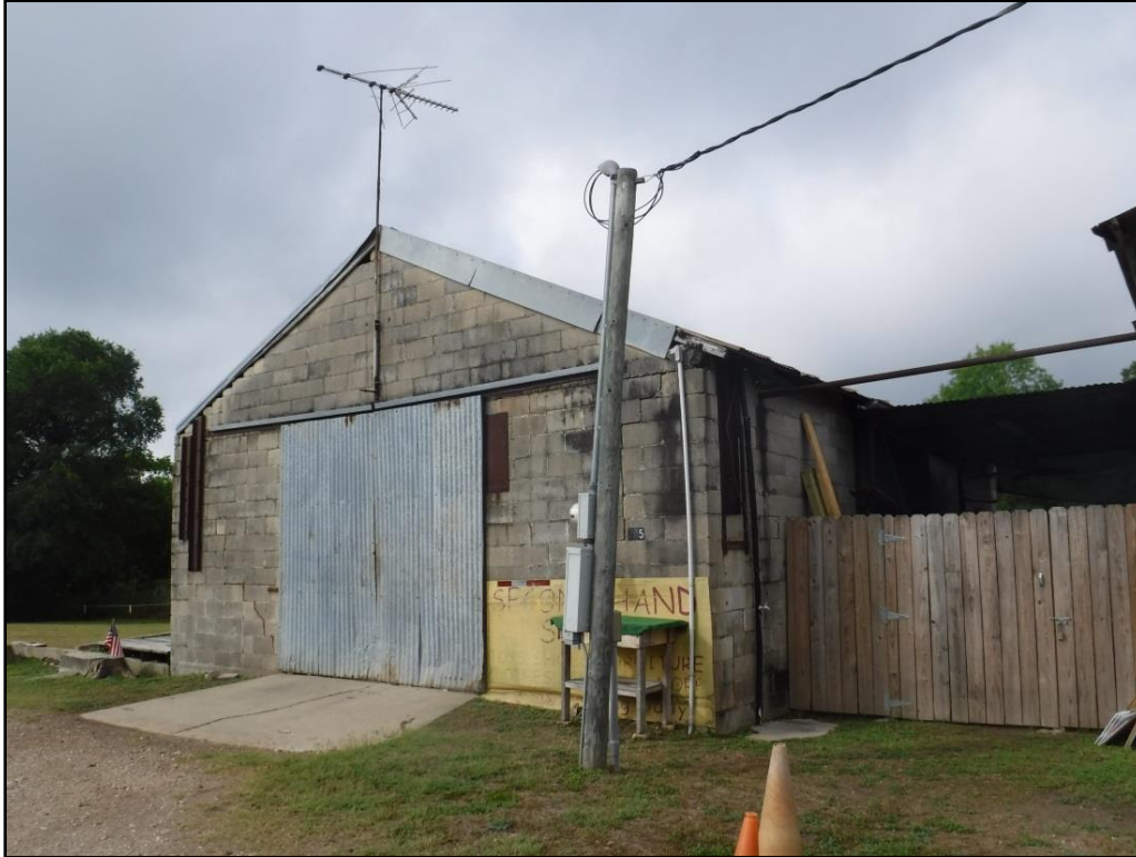
Figure 5-43. Northwestern and northeastern elevations of Historic Resource 3, facing south.
