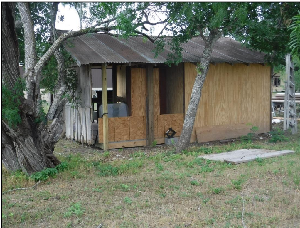
Figure 5-47. Northwestern elevation of Historic Resource 5, facing south-southeast.
