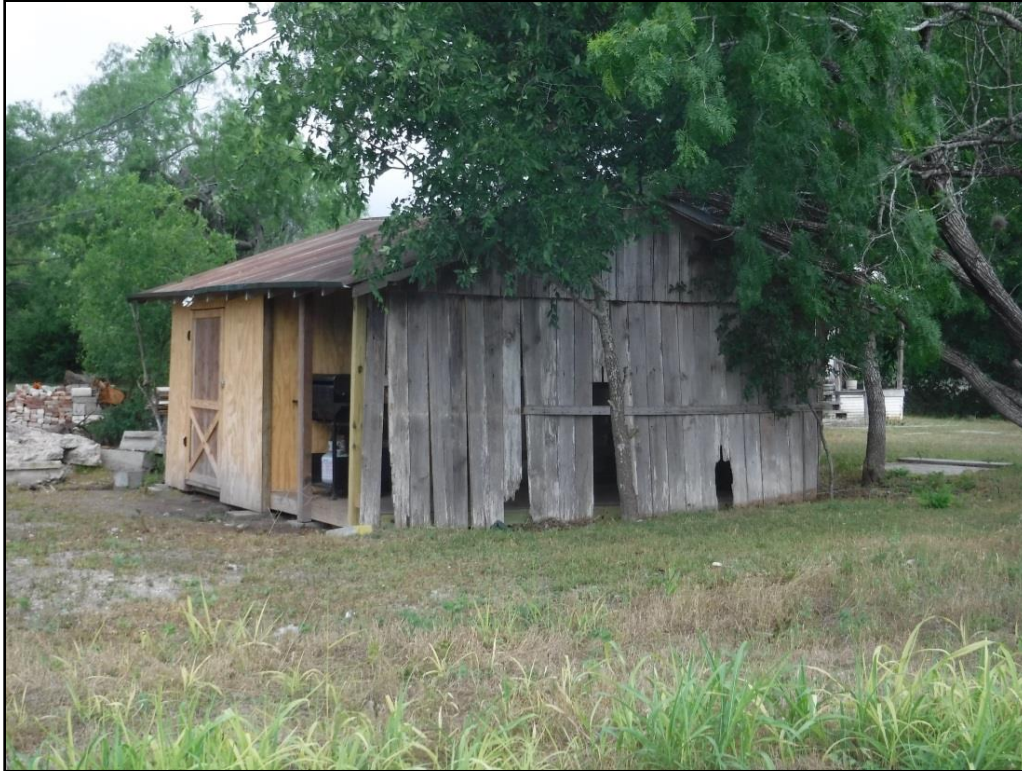
Figure 5-48. Northeastern and southeastern elevations of Historic Resource 5, facing west.
