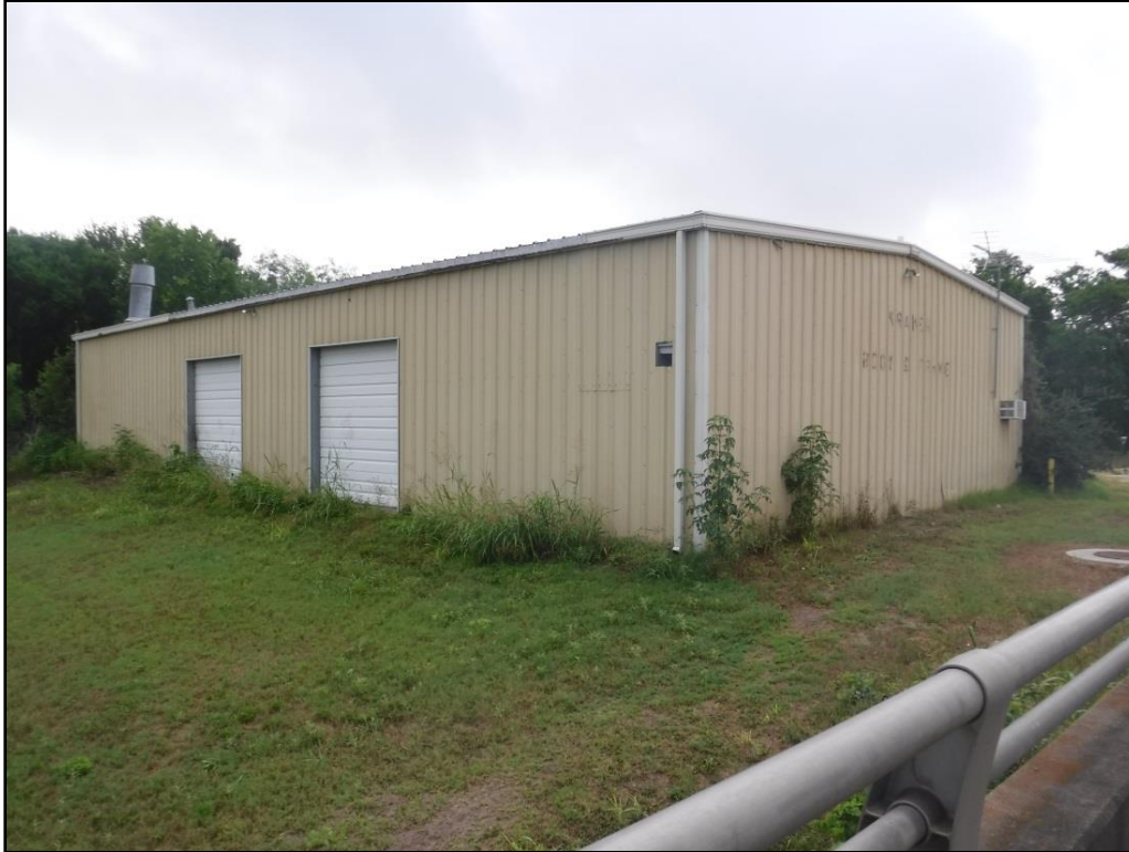
Figure 5-40. Southwestern and northwestern elevations of Historic Resource 1, facing east.
