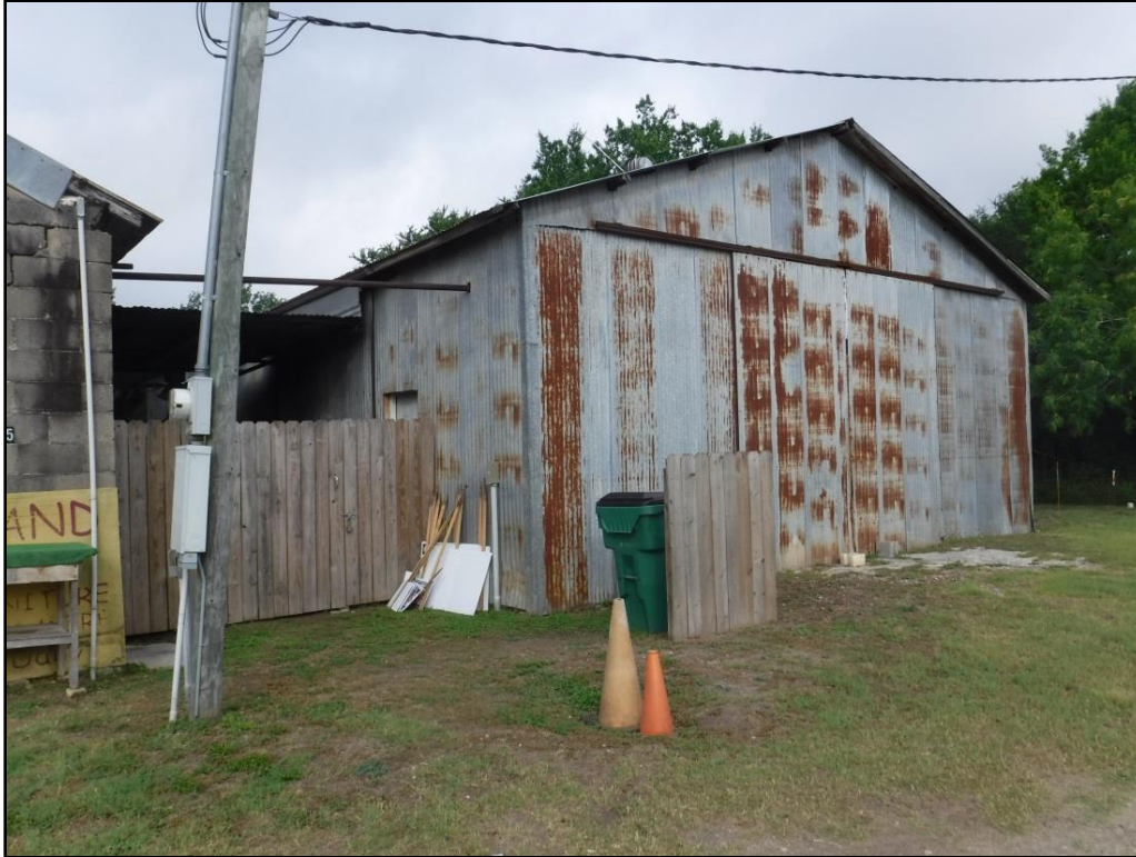
Figure 5-42. Northeastern and southeastern elevations of Historic Resource 1, facing west.
