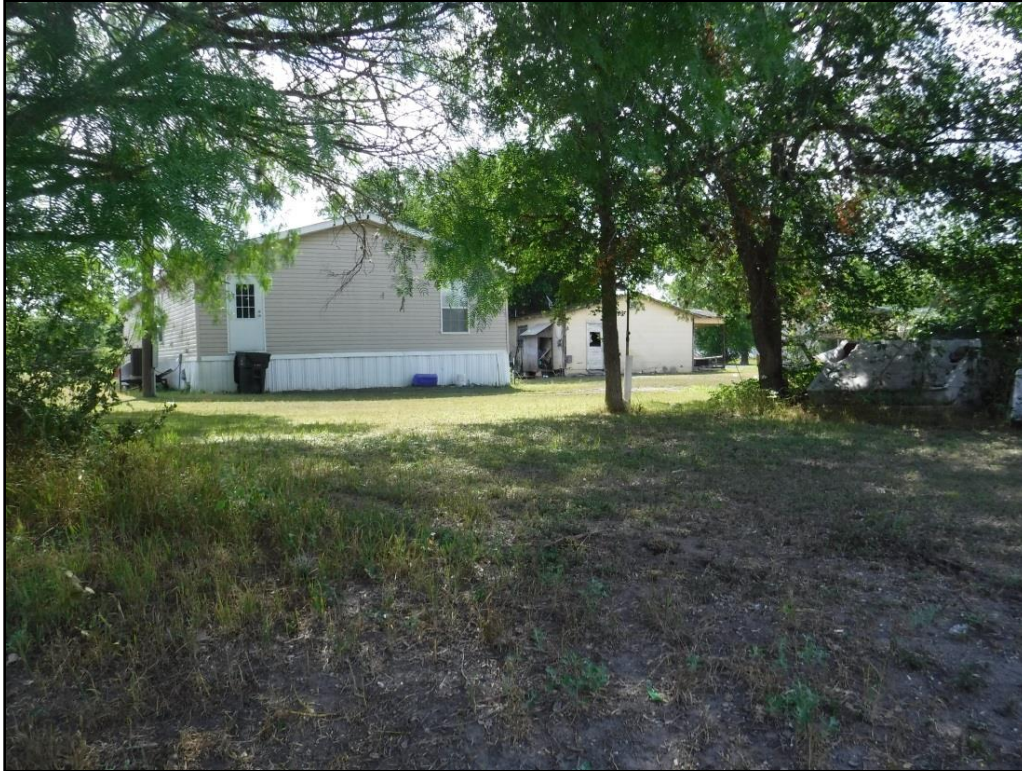
Figure 5-38. Modern mobile home located to the northwest of Historic Resource 6 (background), facing east.
