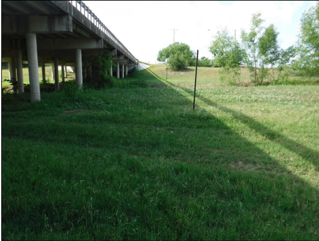
Figure 5-4. Buried AT&T line along the western side of US Highway 181; facing south.
