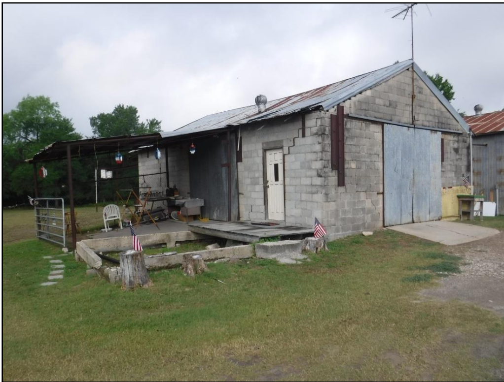
Figure 5-44. Northeastern and southeastern elevations of Historic Resource 3, facing west.
