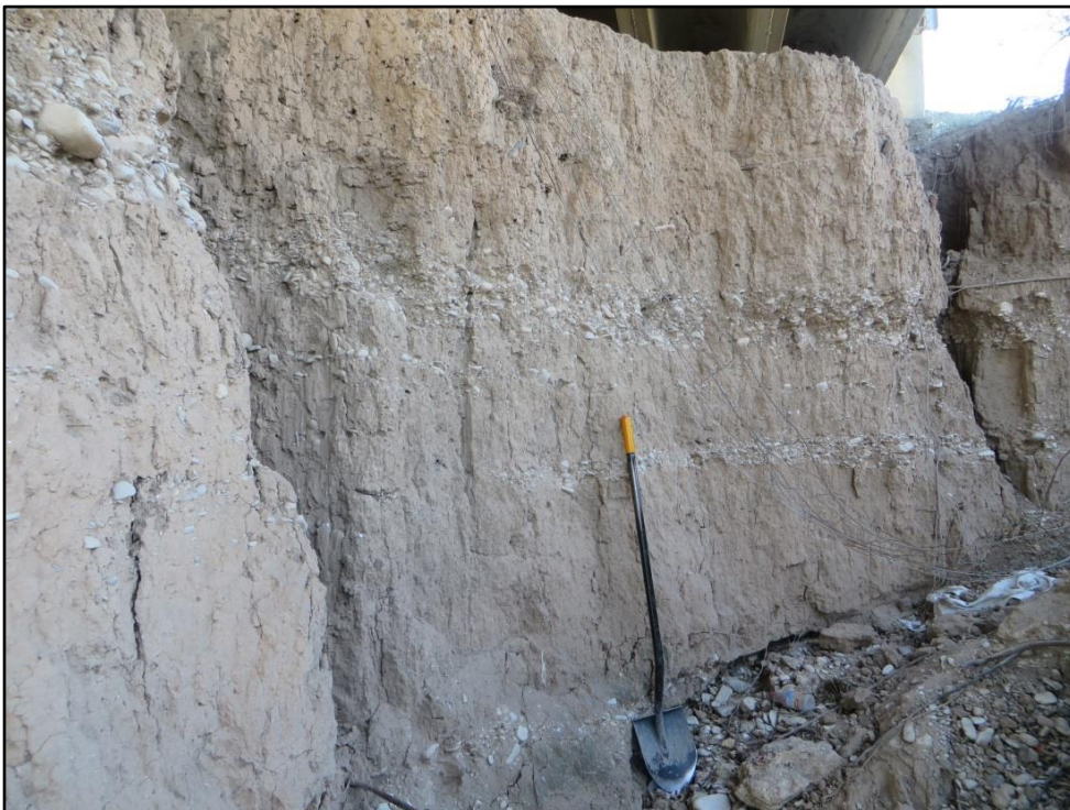
Figure 6-14. Erosional soil profile beneath the F.M. 380 bridge, facing west. Shovel measures 140 cm long for scale.
