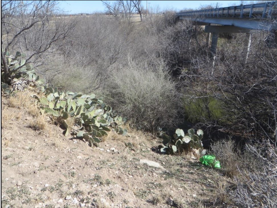
Figure 6-10. Decent (50 to 90 degree angle) into river channel, facing east.
