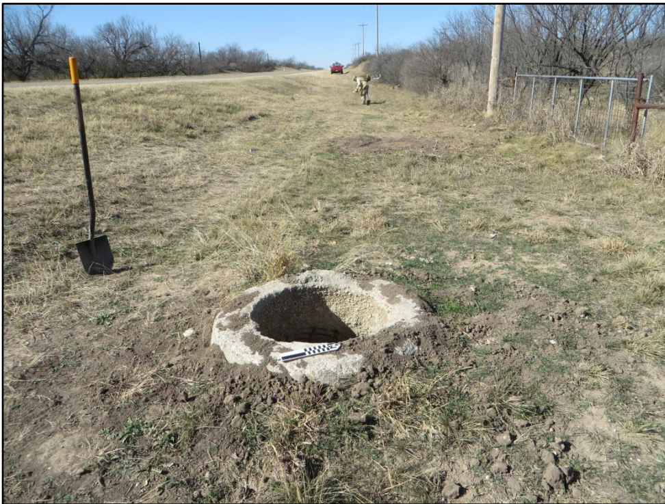
Figure 6-5. Abandoned manhole utility with modern manhole cover in background, facing west.
