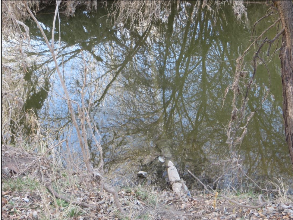
Figure 6-17. Existing pipeline within Concho River, facing east.
