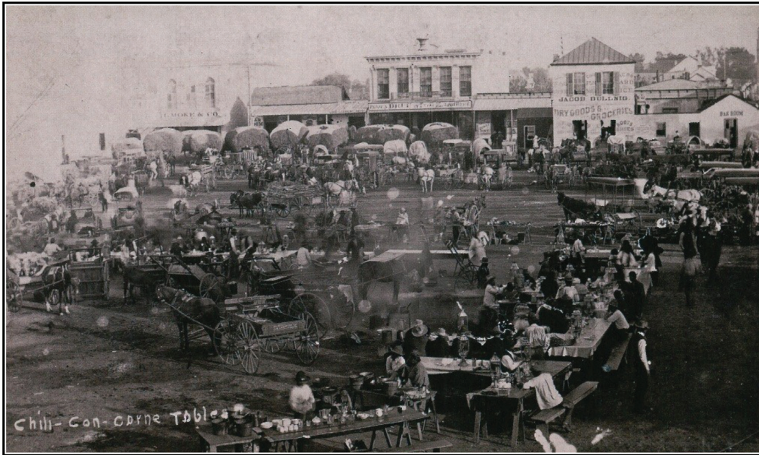
Figure 4-6. Plaza de Armas filled with vendors, ca. 1875-1885, view facing north (image from Steinfeldt's San Antonio Was [1978:44]).
