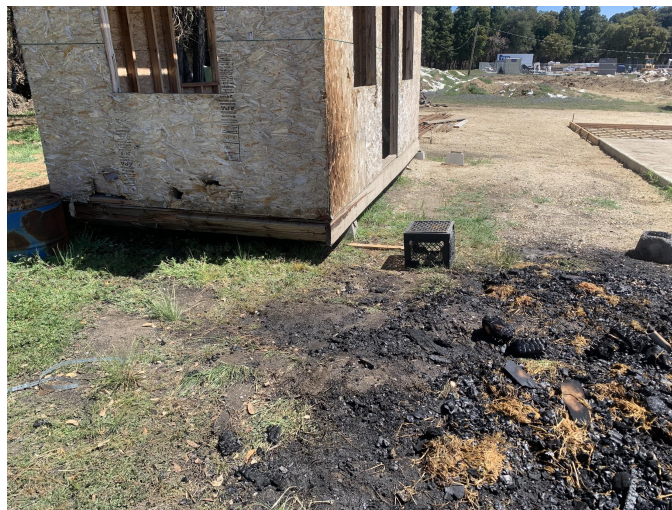
Figure 6.3: Shed surroundings after test
