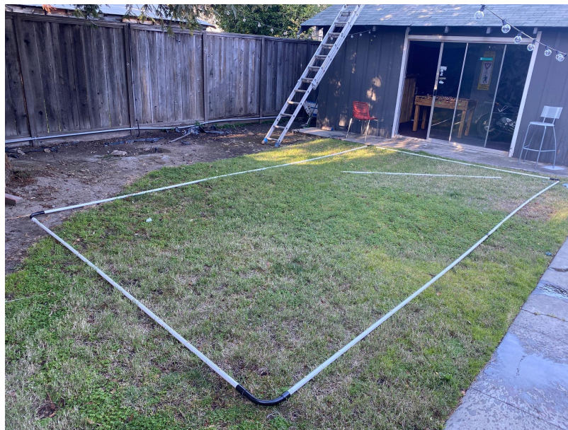
Figure 5.6: Full pipe set up
