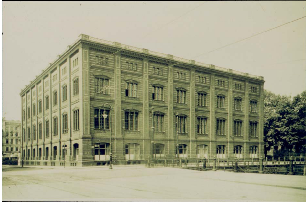
Fig. 35 Image of the Bauakademie
