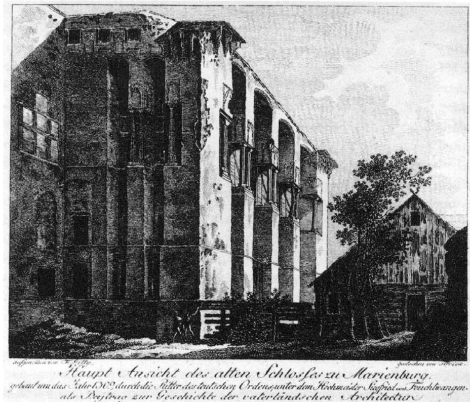
Fig. 23 Image View of the Exterior of the Chapter House of Marienburg 1794- 76
