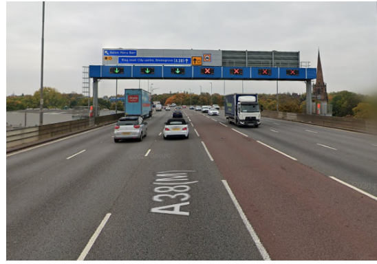
(b) Electronic overhead signs
