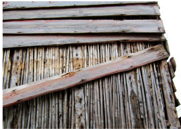
Figure 2. Use of reed for wall construction: palheiro in Leirosa [13].
